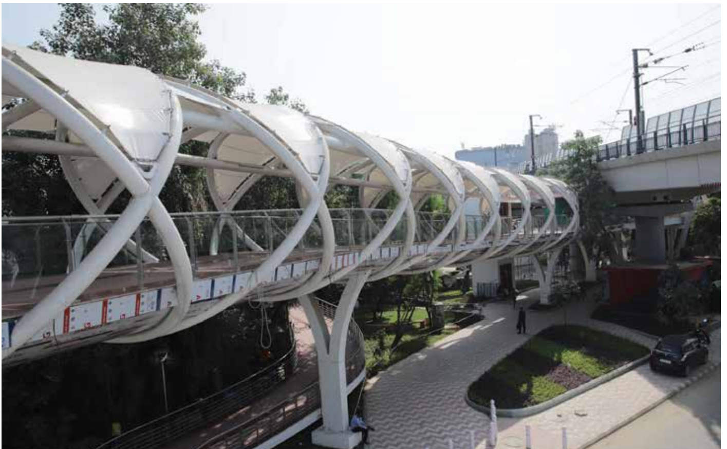
The skywalk and a landscaped footpath create a pedestrian-friendly environment at one of the busiest nodes in Delhi.
