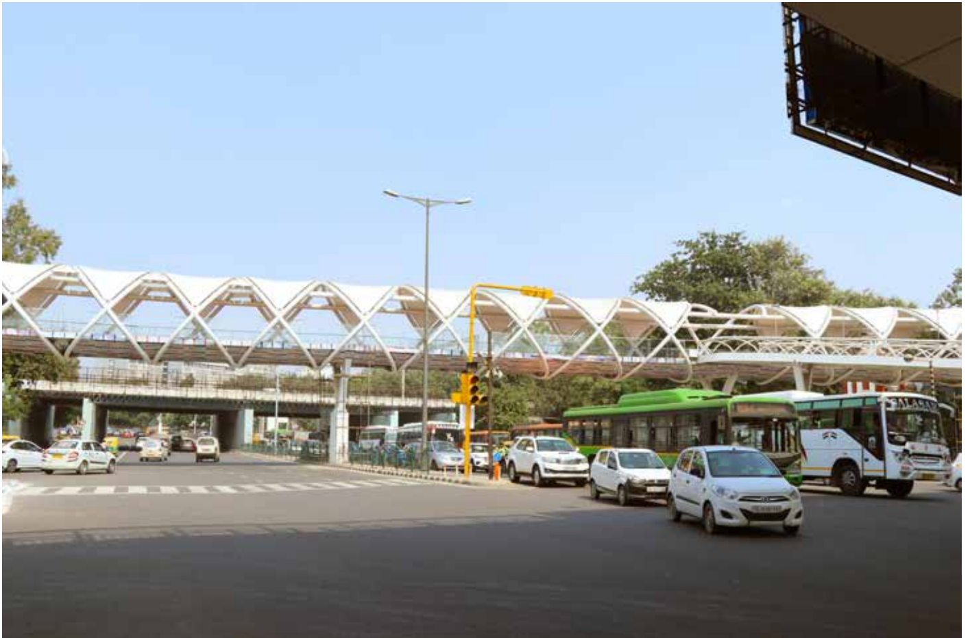
The unique criss-cross boot-lace trusses make the skywalk instantly recognisable from a distance.
