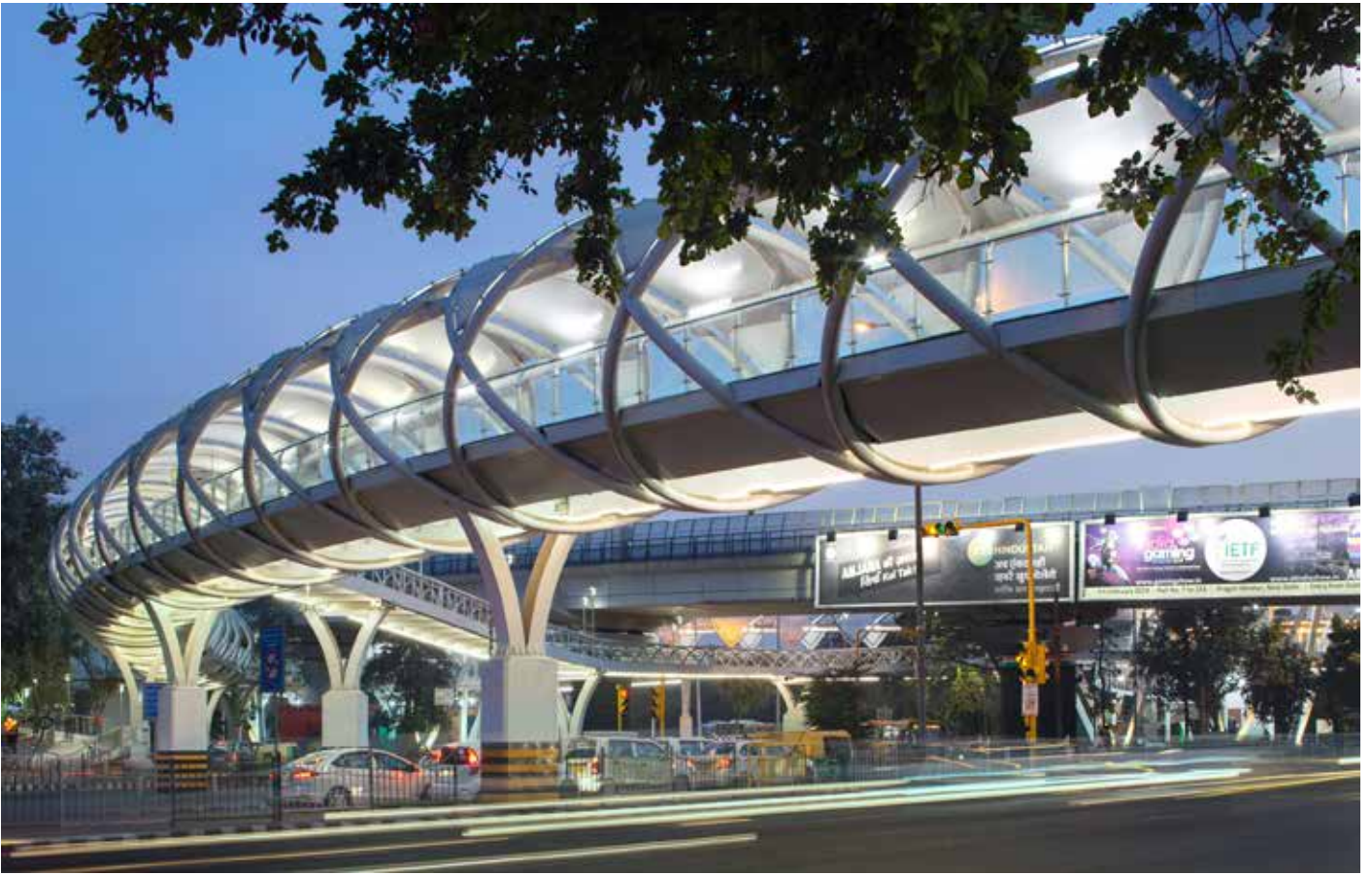
The ITO Skywalk solves the problem of pedestrian movement at one of the busiest nodes in New Delhi, and its unique form is a design and engineering marvel that acts as a significant landmark in the city.
