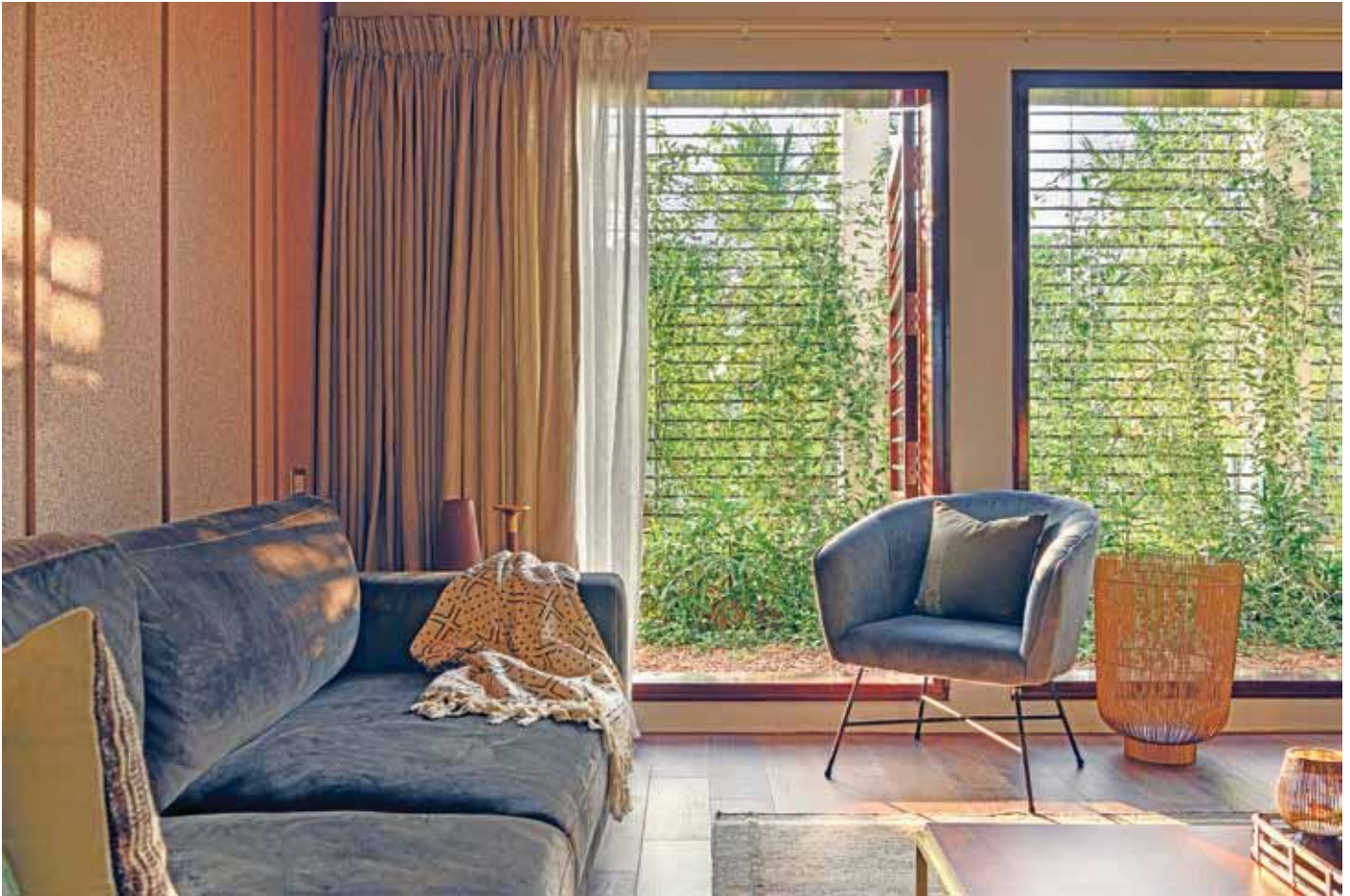
Figure 6: Western sunlight been filtered using double skin structure and vegetation (Source: Author)
