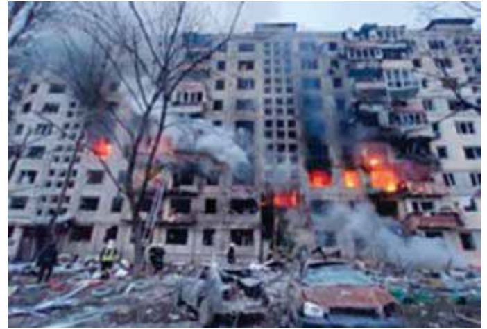
Fig.3: High-rise apartment damaged by shelling in Kyiv, Ukraine on 14 March 2022 (Source: Retrieved, January 15,2023 from https://www.reuters.com/ )
