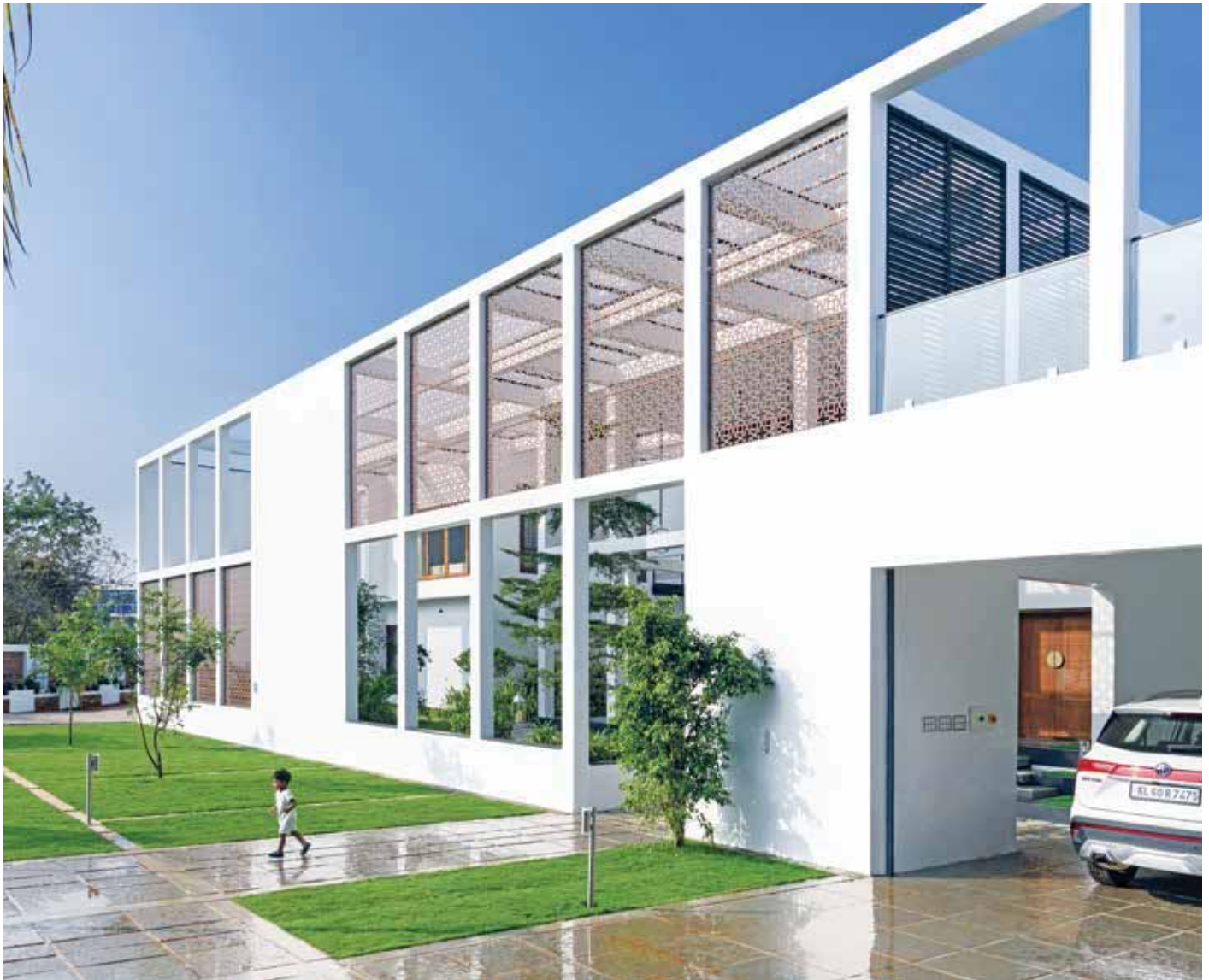
Figure 1: The façade is the second shell that creates a chuttu verandah around the home. (Source: Author)
