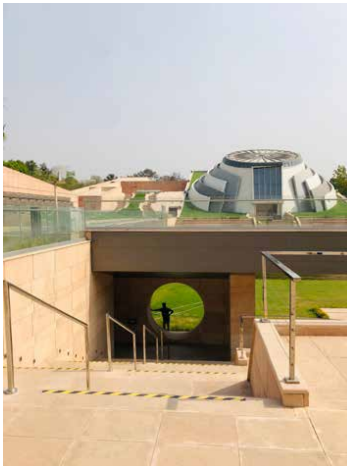
View of Building II as seen from Building I Court
