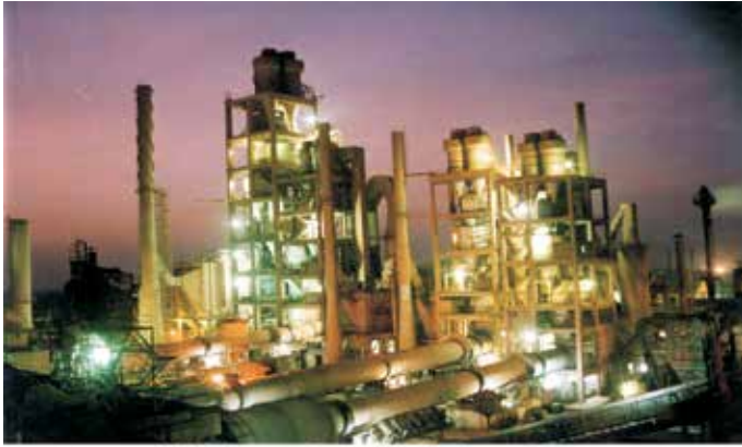
J.K. Cement Ltd., Nimbahera Plant (Grey Cement)
