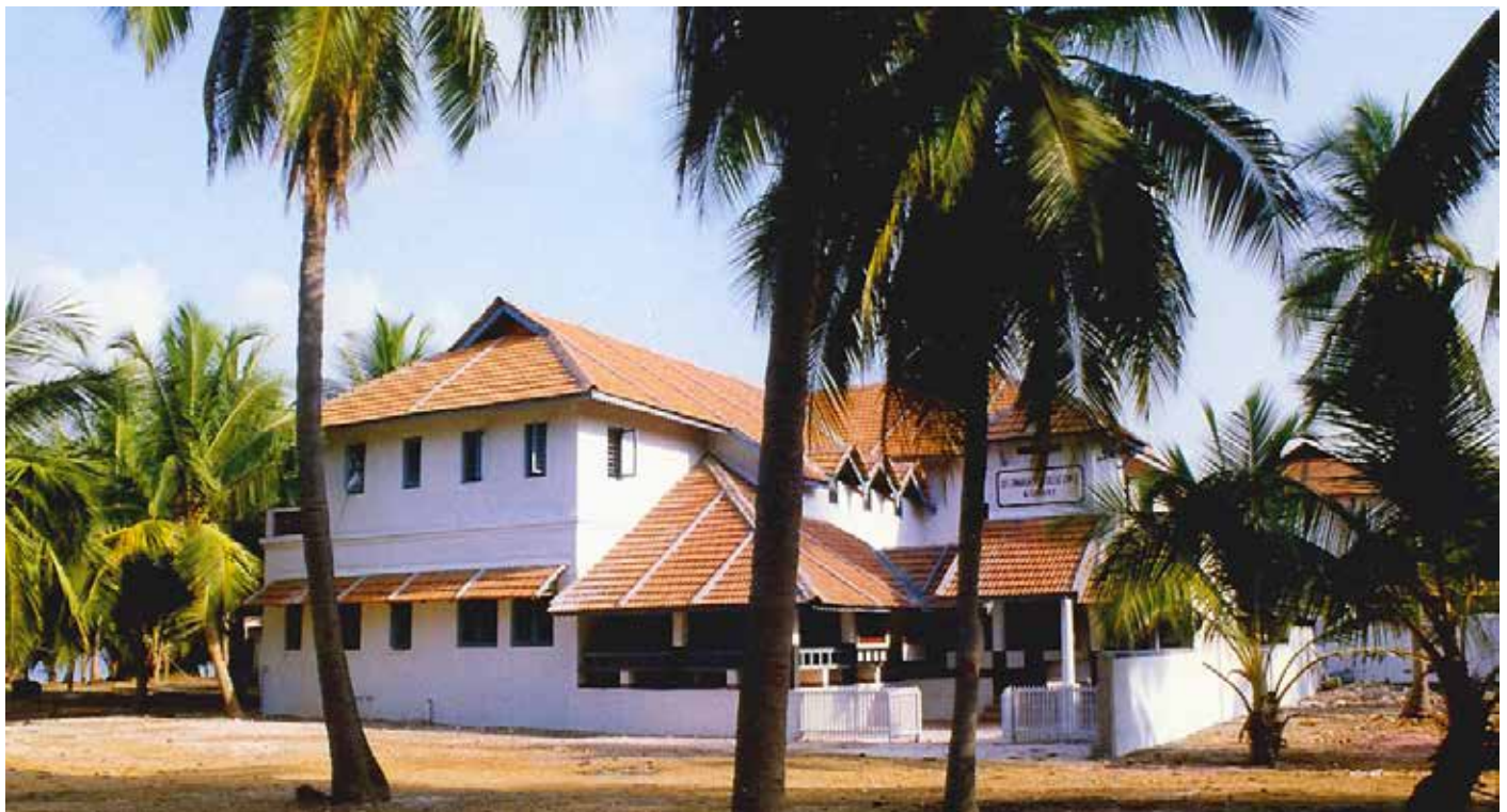
Open land, open approaches, without roads and saving every tree. Jawaharlal Nehru Junior College, Kadmat Island, Lakshadweep. (Source: K.T.Ravindran)
