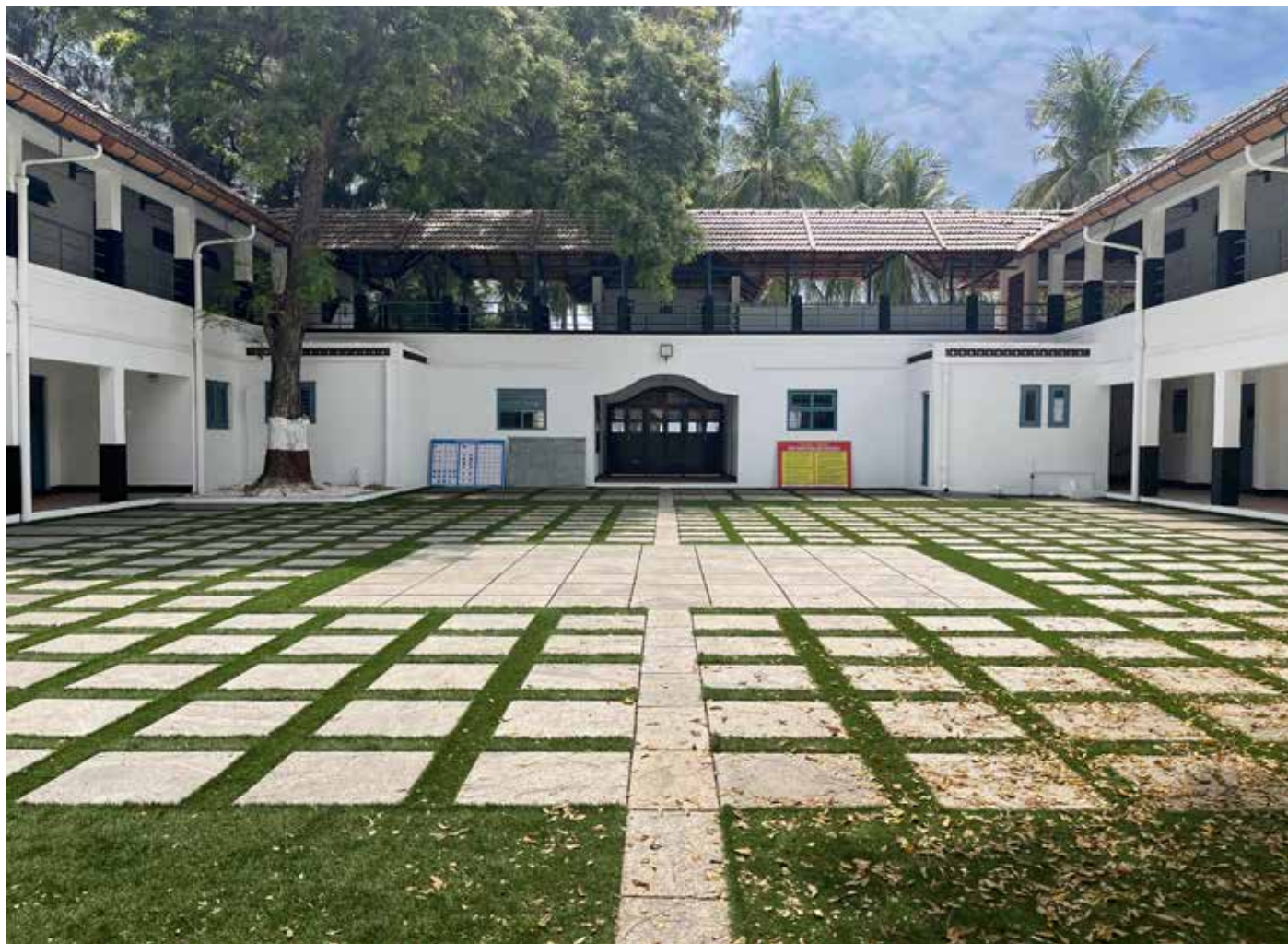
In land scarce island a TB sanatorium was restored, added to create a modern residential Junior College. Jawaharlal Nehru Junior College, Kadmat Island, Lakshadweep. (Source: Akshaya K)
