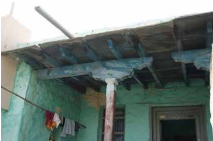
Fig 3: Stone slab roofing in Bukkasagara, Hospet, Karnataka 2019 (Source: Author)
