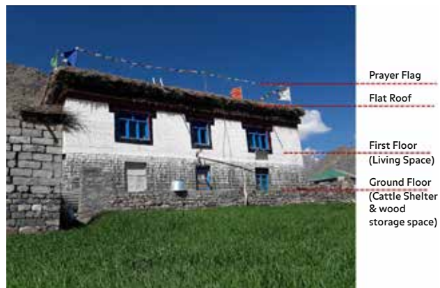
Figure 5: Mud structures showing Spitian style and their components (Source: Author)
