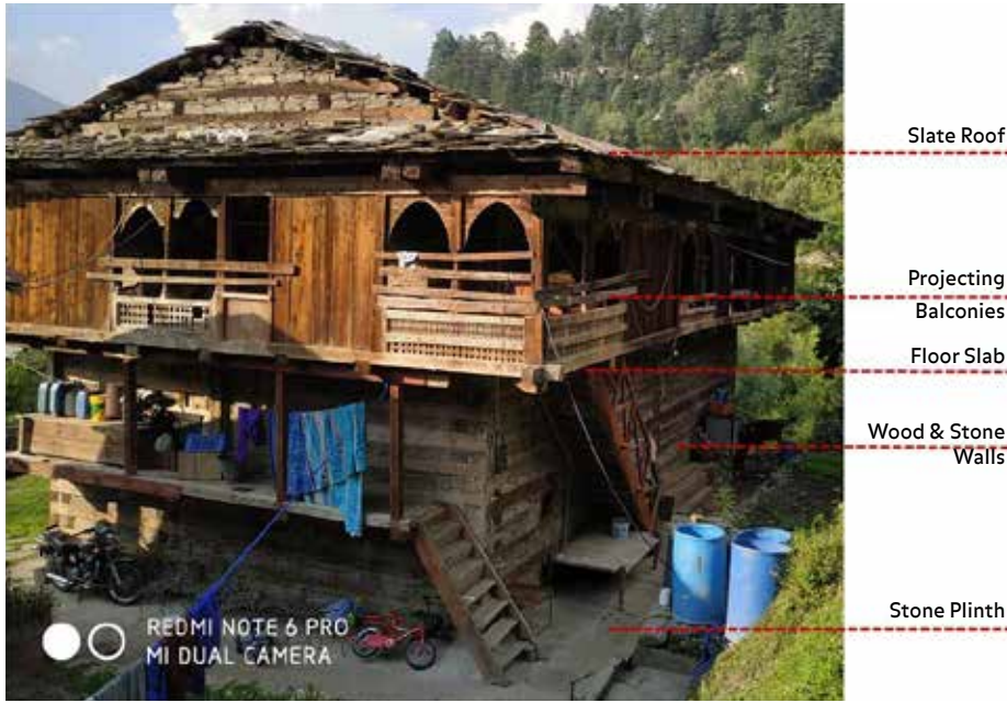
Figure 1: Kathkunni structure with their components (Source: Author)
