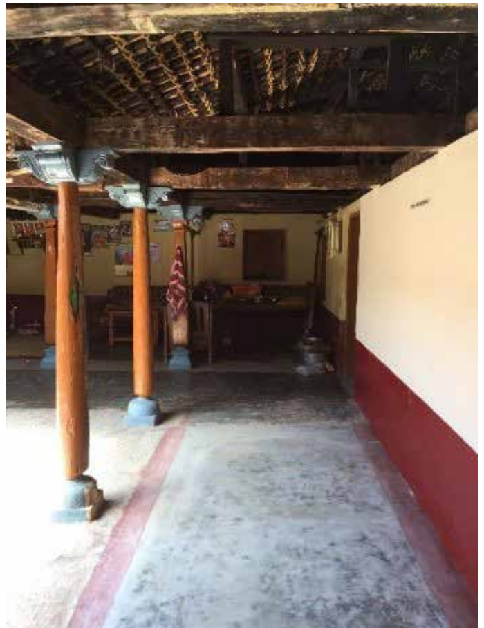
Fig 4: Timber truss with split bamboo battenings, tied with rope, Aretipur, Mandya, Karnataka 2018 (Source: Author)
