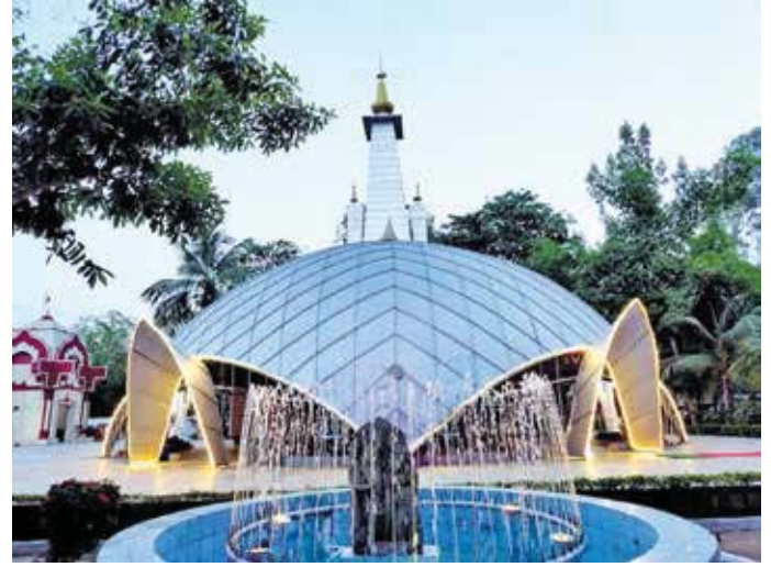
EME Temple is an outstanding modern structure, with a geodesic dome clad in aluminium sheets.
