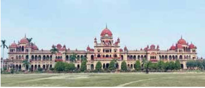
Fig. 9 : Façade adorned with elements and features of traditional architecture of Punjab in Khalsa College, Amritsar Source: Corresponding Author
