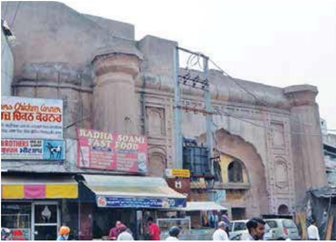
Figure 4: Shops and Hoardings eclipse Ram Bagh Gate Source: https://www.tribuneindia.com/news/archive/amritsar/old-gates-around-walled-city-cry-for-attention-261302
