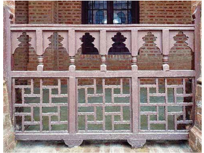
Fig. 4 : Traditional geometrical lattice work in the railing design in Khalsa College, Amritsar, Punjab Source: Corresponding Author
