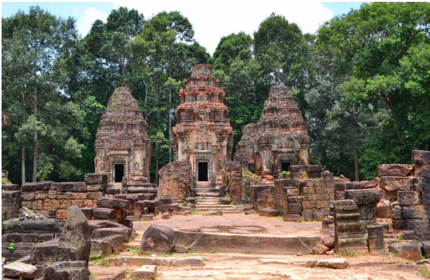
Structures in the vicinity.
