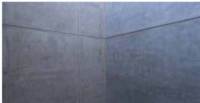
Stabilised lime finish to replace paint.
