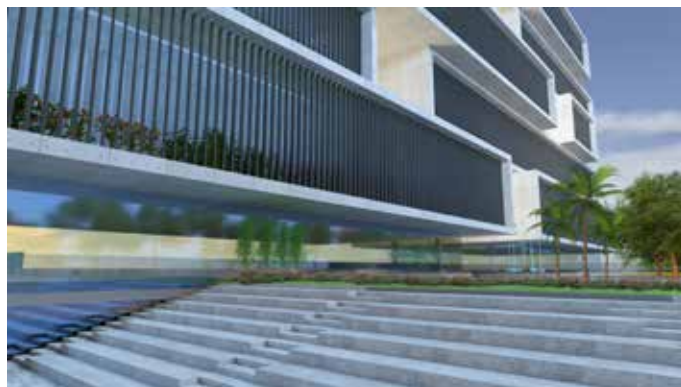
Figure 4: Vertical Louvers on East & West Side
