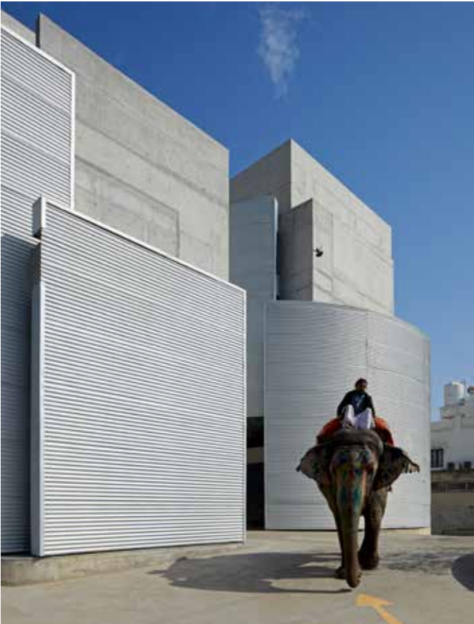
Open Door, Ahmedabad. A composition of openable corrugated Galvalum (steel) and fixed raw concrete planes.
