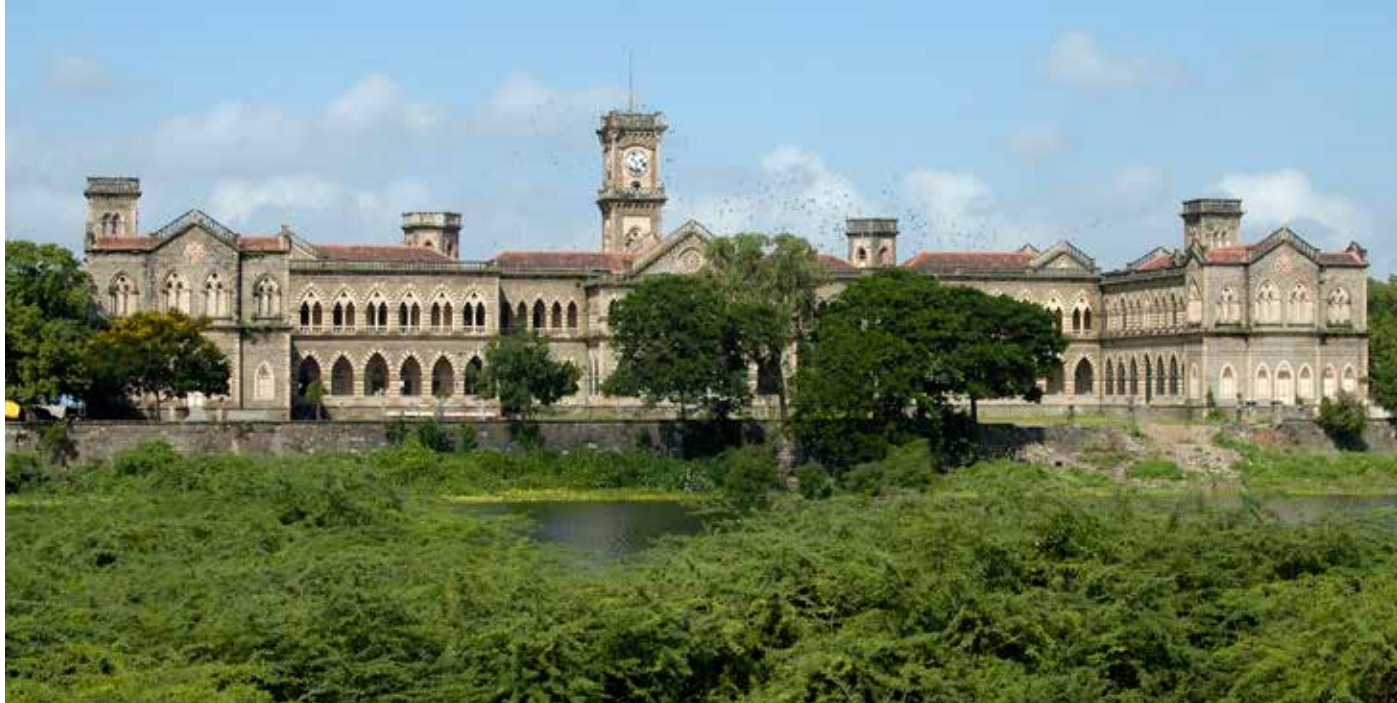
Sangram Singh School, Gondal. Originally slated for demolition after the devastating 2001 earthquake, the studio instead intervened and retrofitted the largest heritage building in Gujarat. Budget - efficient and low cost.
