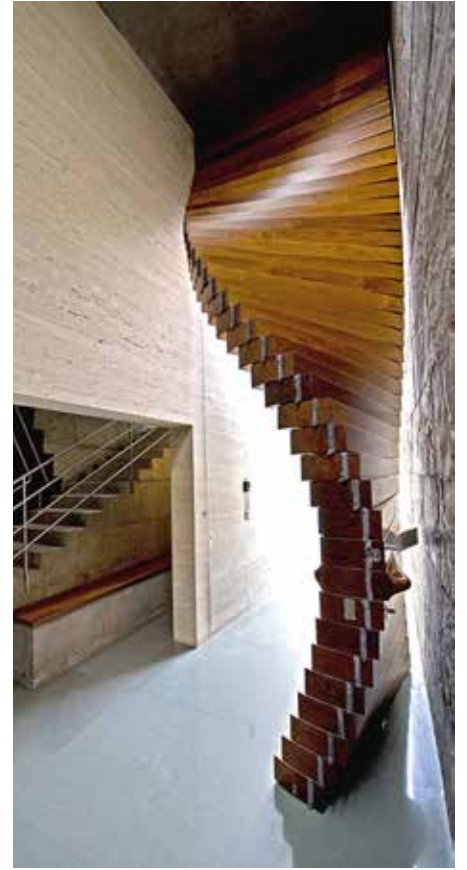
Curtain Door: 40 Logs of wood tied with a string, opening in a sinuous curve.
