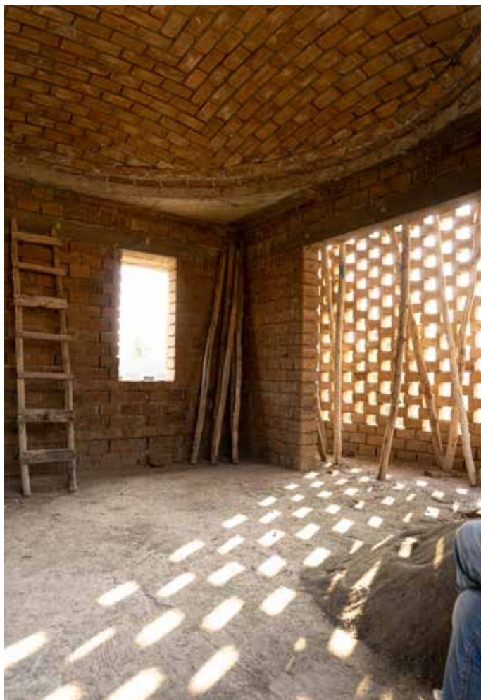
Geodesic dome with CSEB bricks.
