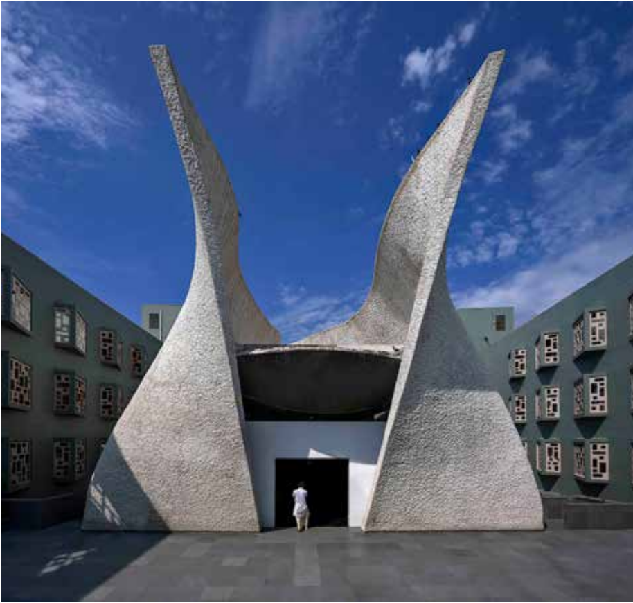
Man-made God, Ajmer. Square in plan, the temple gently morphs into a sinuous volume, signifying an open interpretation of religion.
