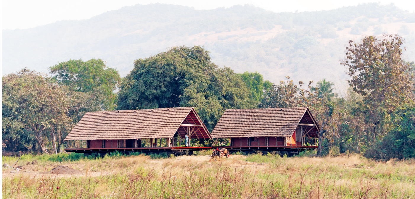
The two linear bamboo and timber structures at GoodKarma Farms, Alibaug. The larger unit is a common processing area, and the smaller unit is an ensuite room.
