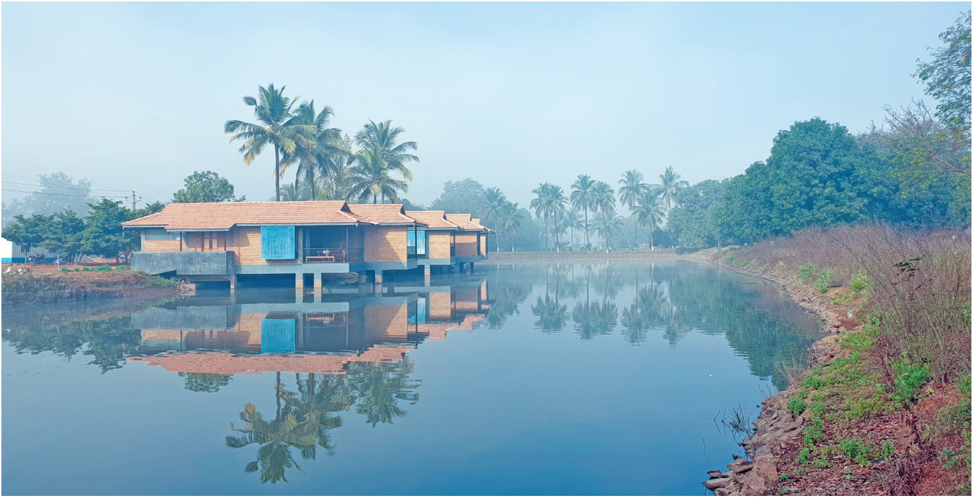
The pondhouses at Saguna Baug Agro Tourism Centre, Neral, Maharashtra. The structures are made using CSEBs (Compressed Stabilised Earth Blocks).
