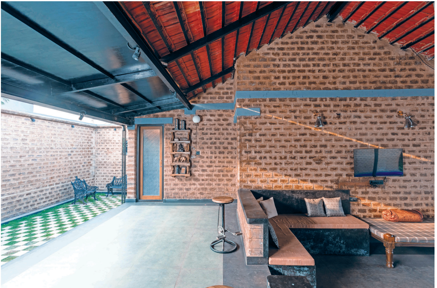
The Nirvana Joy farmhouse, which is an annexe of the former, is on the banks of the river Bhadsa in Khadavli, Maharashtra. The project is done using CSEBs
