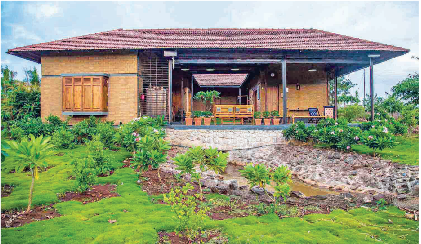
The Nirvana Peace farmhouse, on the banks of the river Bhadsa in Khadavli, Maharashtra. The project was done using CSEBs.
