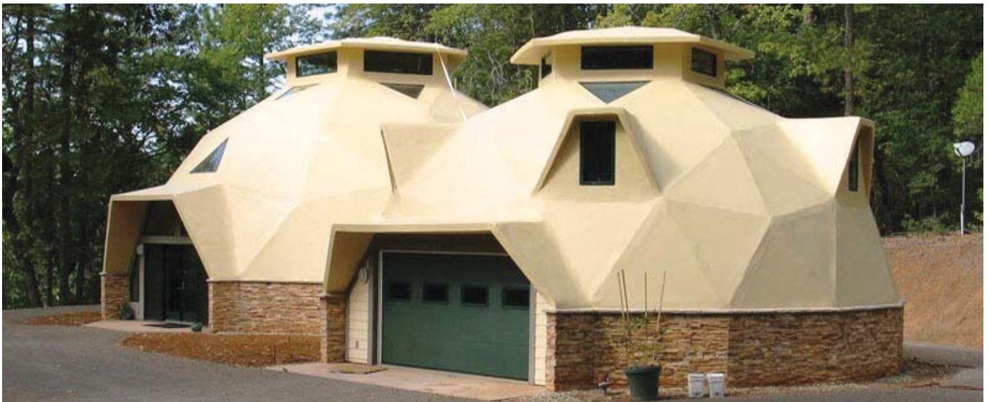
Fig. 6: Geodesic Dome-Shells with Concrete Panels
