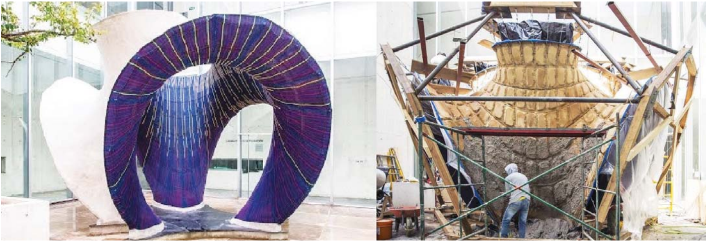
Fig. 8: Knit Candela shell: Finished and Under-construction
