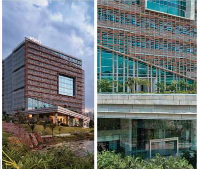
Some portions of the façade do not have a second skin and are inset by 2m into the building for glare and heat protection
