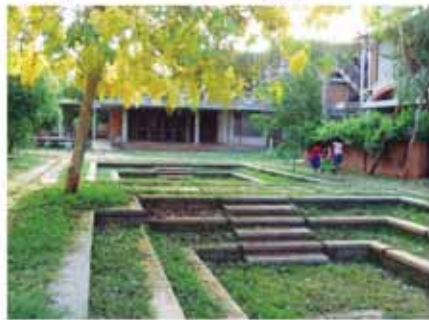
The central courtyard - rainwater harvesting and percolation
