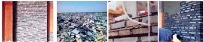
02. WASTE CUDDAPPAH WALL - Factory waste, cuddappah trimmings used as walling in rain exposed zone
