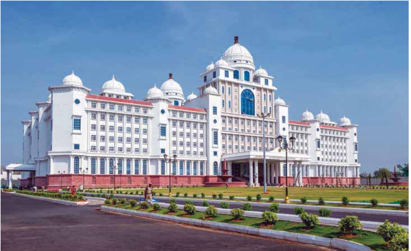
Fig. 2: Front View of the Telangana State Secretariat
