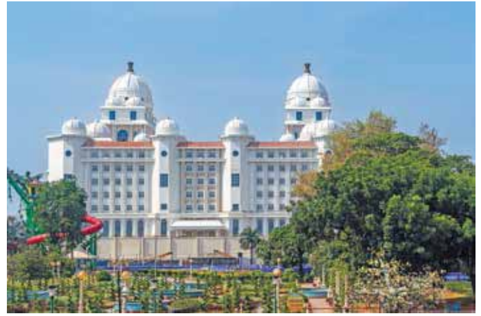
Fig. 3: Side View of the Telangana State Secretariat
