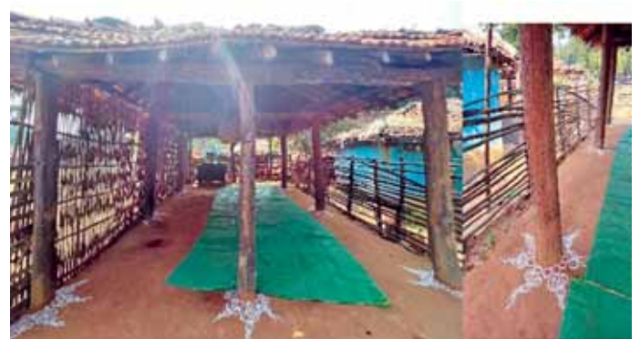
Figure 8: Ghotul at Mendha village with bamboo walls, compound walls as well as base of the support decorated with rangoli Source: Authors
