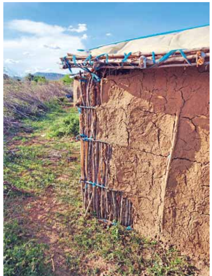
Fig. 10: Cow dung plaster on framework
