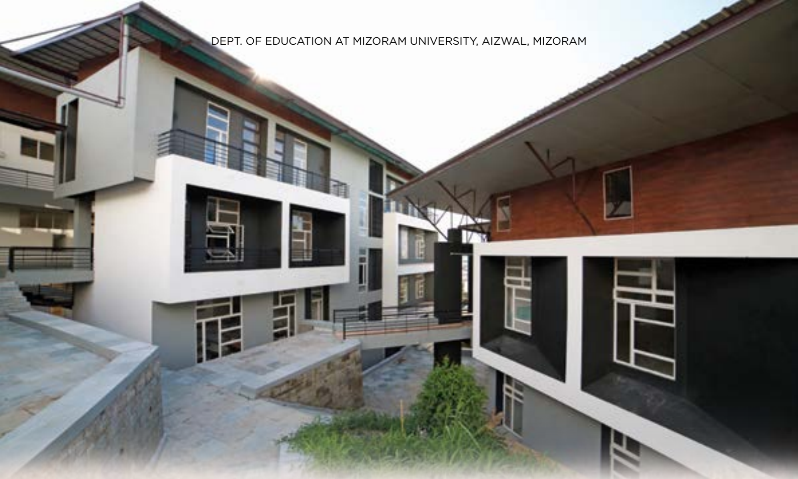
Stairs lead down to the Seminar Hall on the right, and classrooms are on the left.
