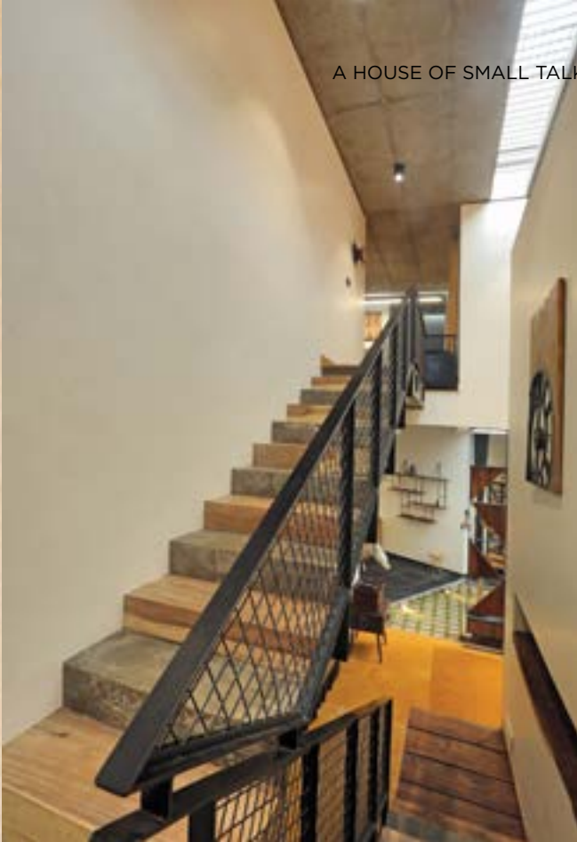
The folded staircase imprints clear lines of alternating exposed concrete and wood with old fashioned steel railing
