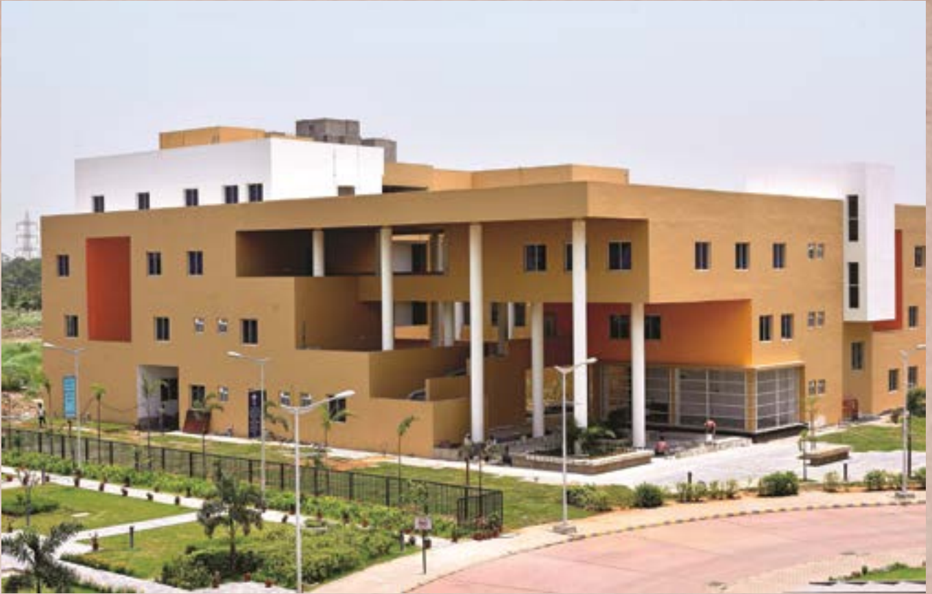
Interplay of solid and void enables effective visual connection and physical continuation of space
