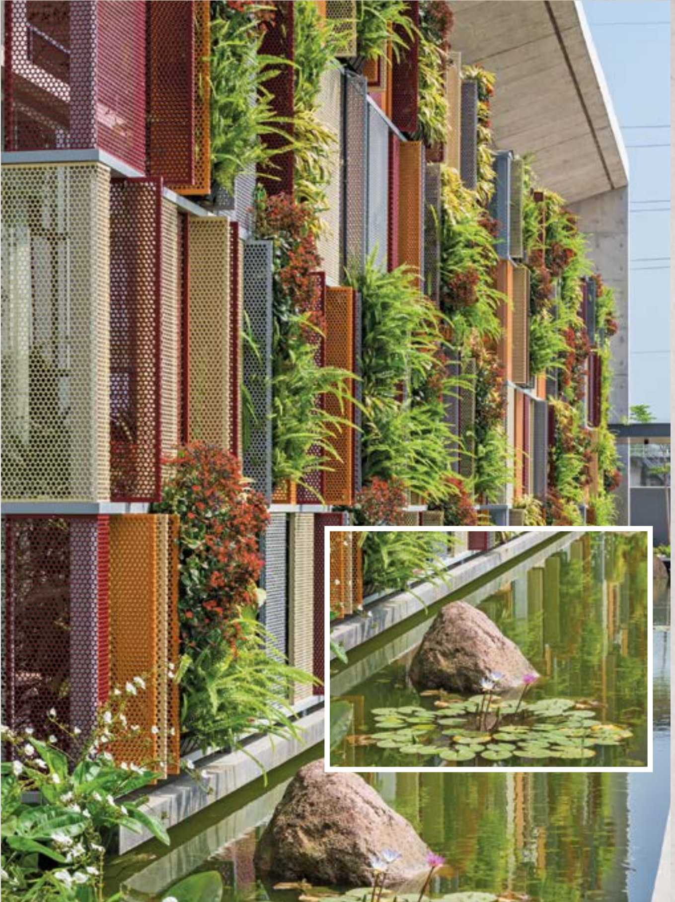
Breathing Wall - A perforated panel's screen on the front facade cuts off the glare in the summer months. The screen is kept at a distance from the main utility areas thus creating small courts.
