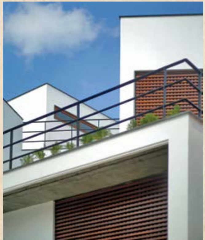
The terpsichorean composition of various volumes creates a layered up-built of the house
