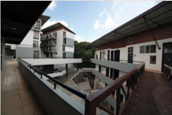
Lower courtyard looking towards the South, Building on the West shades the courtyard from the harsh afternoon Sun.
