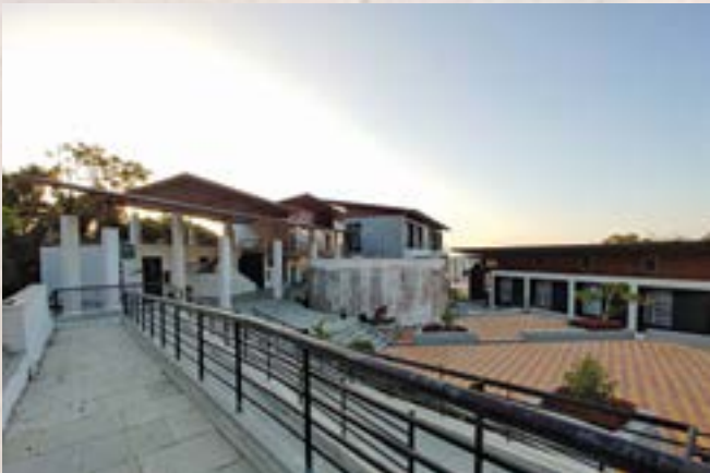
ramp entry from the road, looking towards the main entrance canopies
