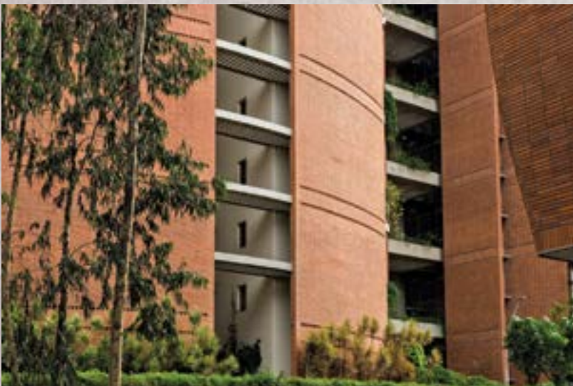
Photograph of Tower 1&2, March 2017
