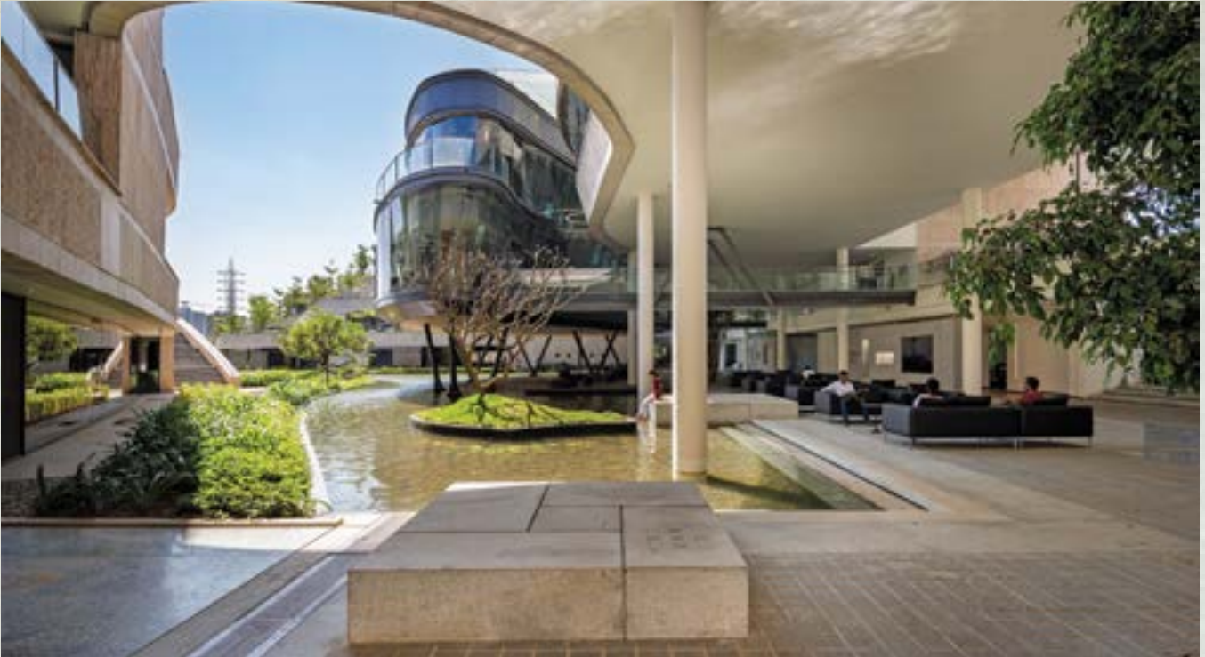
Central spine with Managing Director's Office Block floating above water
