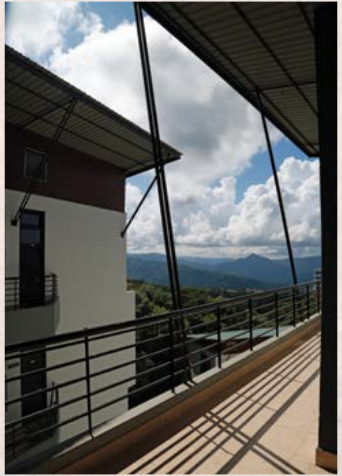
Views of hills beyond from the verandah. Deep overhangs protect from the rain.
