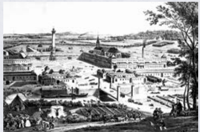
Fourier's phalanstery was a gigantic building housing a co-operative commune of 400 families engaged in agricultural activities. Illustration by Charles-Francois Daubigny, 19th Cent. Architecture in the service of an idealized, rational society. Illustration for "Fool's Paradise".
