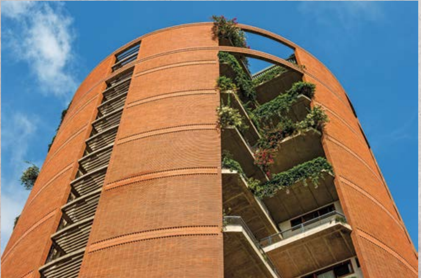
Photograph of Tower-1, March 2017
