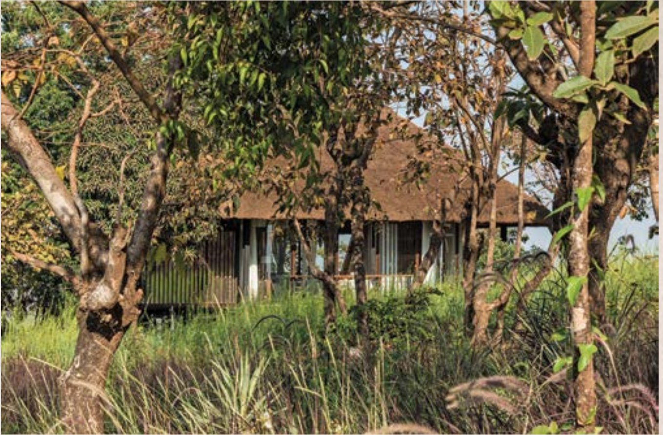
The spatial composition in an otherwise traditional tropical roof structure lends a sense of softness, sensuality, intimacy and complexity, making it a perfect setting for a retreat into the wilderness of Tala.
