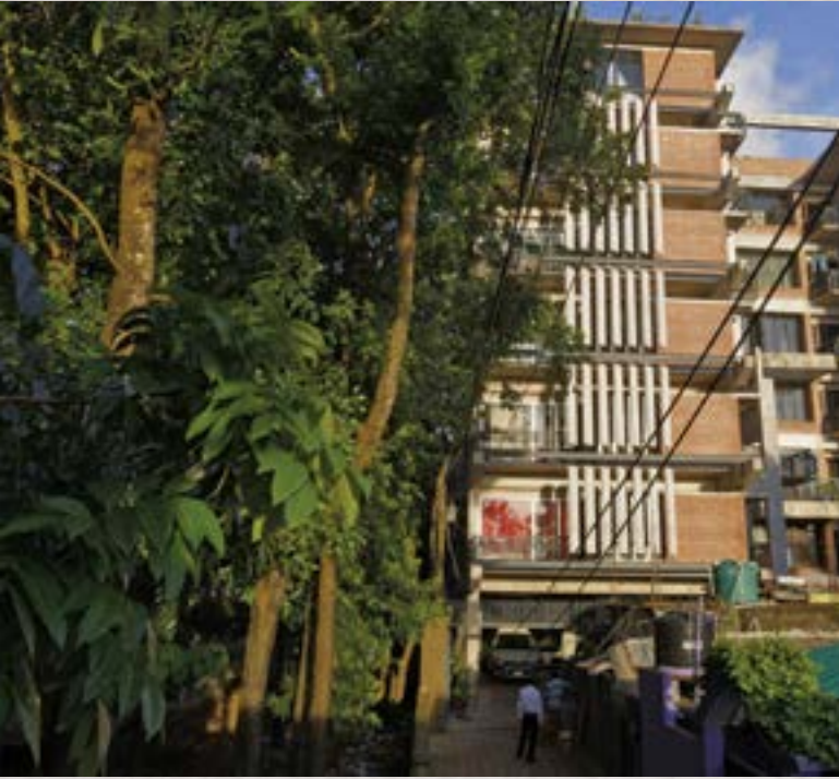
From Entrance North-West
