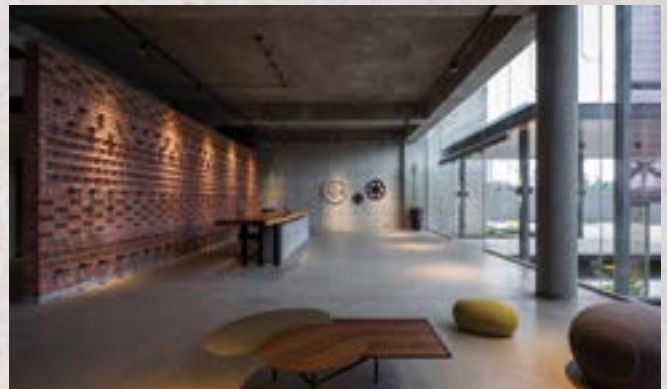
The randomly arranged bricks kept for baking in a local kiln formed the inspiration for this statement wall, the hollow bricks in upper tiers acts as diffusers for the air conditioning duct behind.
