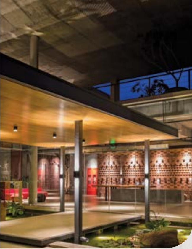
The backwall of the reception draws inspiration from the random stacks of the bricks left for baking in a local kiln. The porosity offered by the hollow bricks in the backwall facilitates air-conditioning and keeps the space light.
