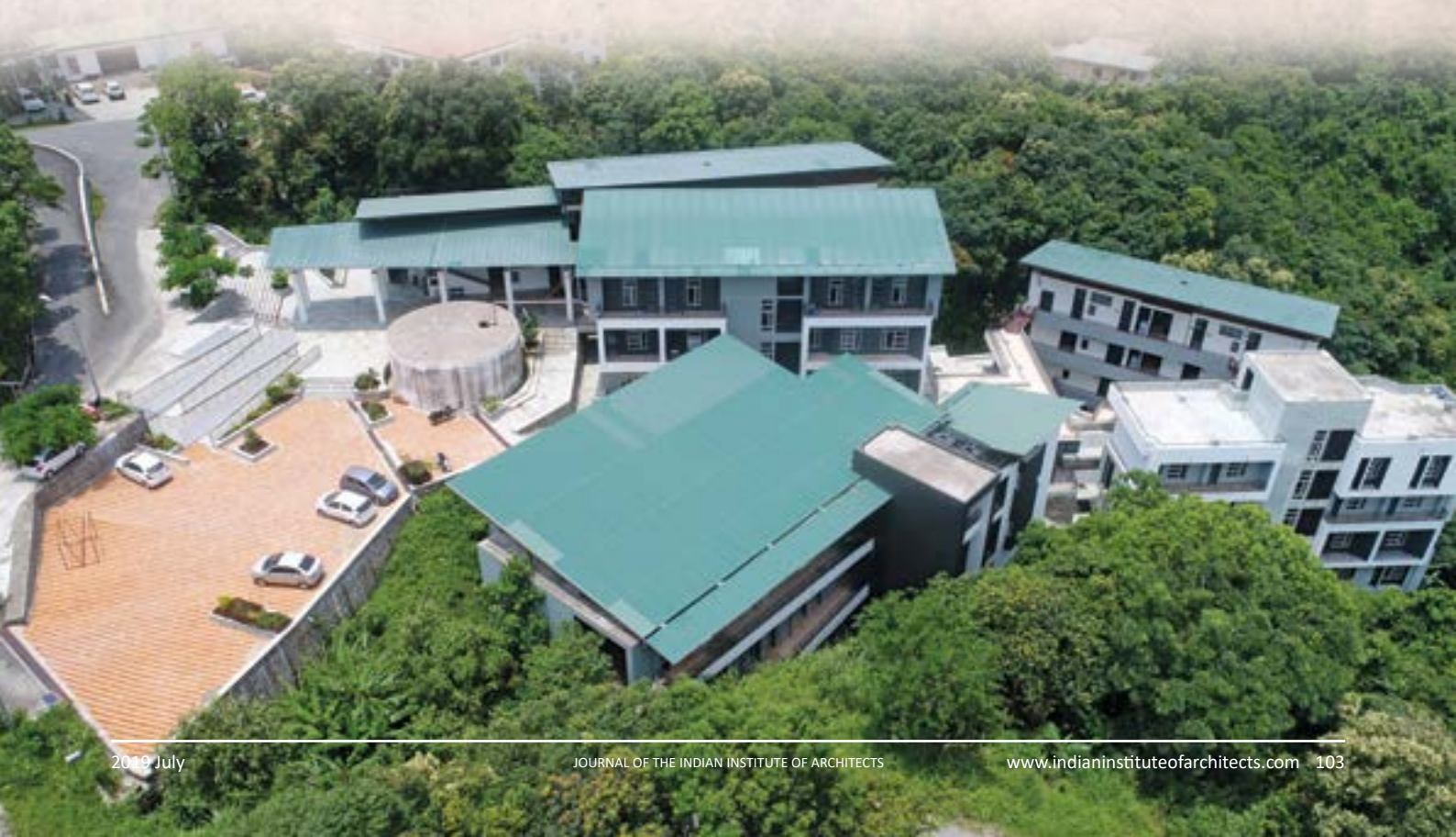
Bird's eye view from the north-east. Buildings are inserted amongst the trees
