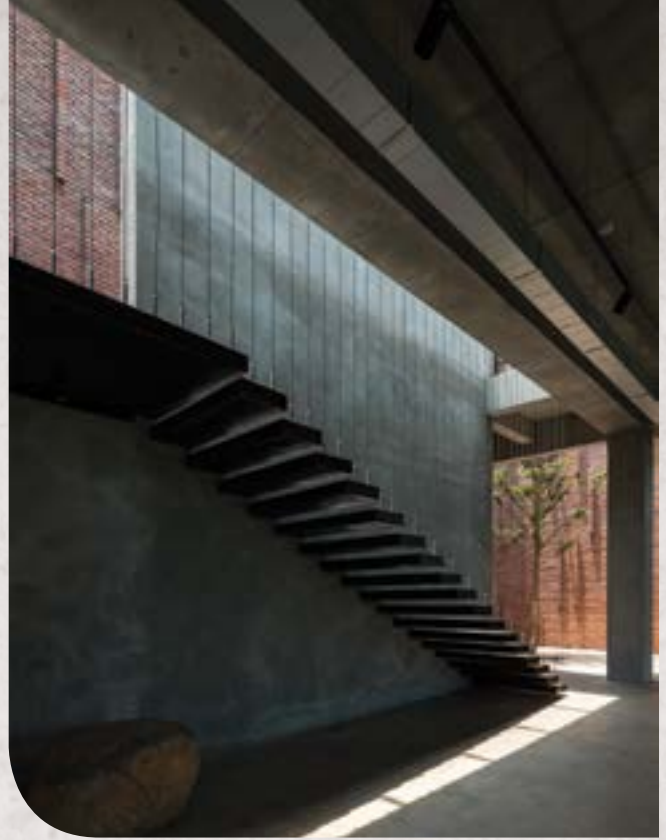
Hanging Stairs - The floating MS staircase imparts the lightness to the circulating areas. The stretched metal ropes in place of staircase railing offer the transparency.
