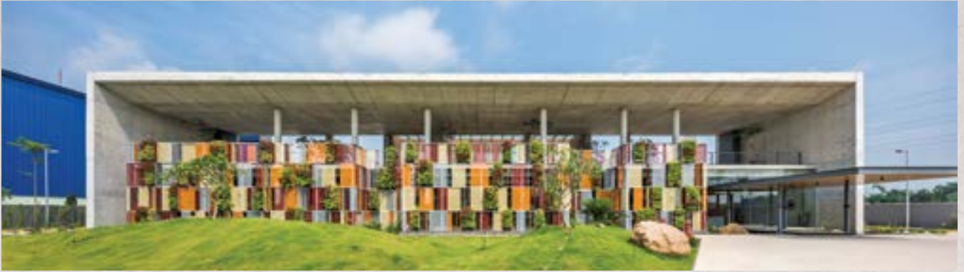
The mass is simple form-finished concrete envelope with a long colorful perforated metal screen adorned with landscape in and out on the front facade cuts off the glare in summer months yet facilitating the air movement.
