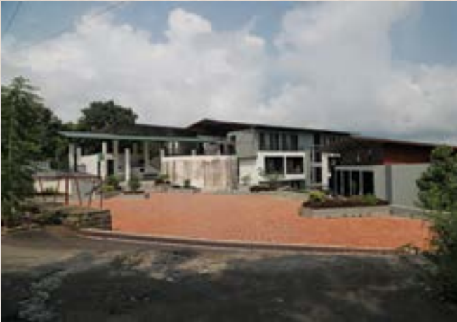
Parking area entry from the road. Main entry canopies on the far left, and existing water tank in the middle.
