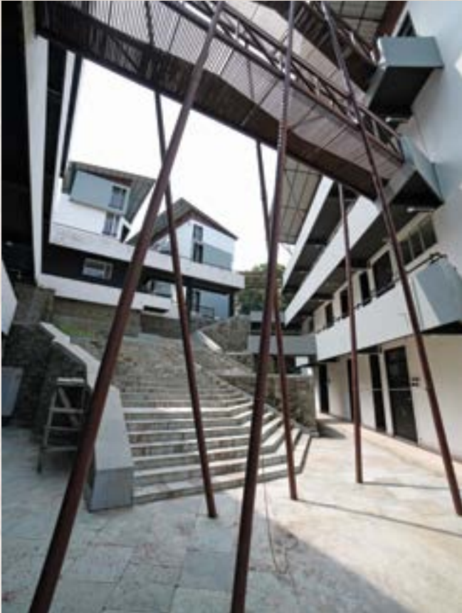
Steel bridge linking the buildings of the lower courtyard. The bridge is made porous to allow breeze to flow through
