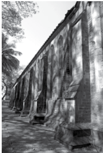
5. External Façade showing masonry & buttresses, Photo: Enoch Rodrigues
