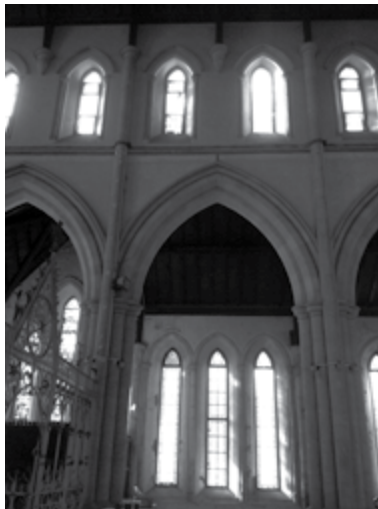
8. Splayed window openings at the Afghan Church, Photo: Author
