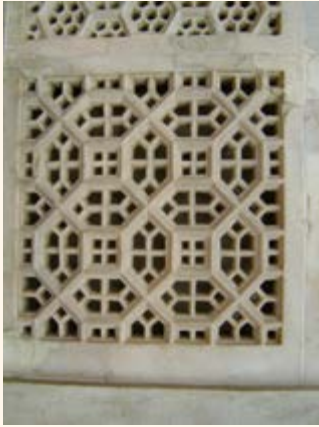
Marble jali panel of Mughal Architecture Agra Fort, 16th century Source: Author
