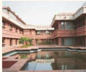
Pond in central courtyard by Raj Rewal's the Parliament Library at New Delhi, 2003 Source: http://ebuild.in/gallery/parliament-library
