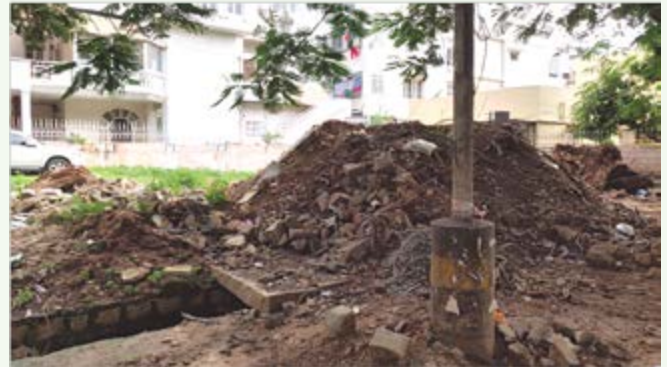
Fig. 2: C&D debris illicitly dumped on vacant sites in Vijayanagar, Bangalore creating poor public realm & blocking sidewalks (Photo by Author on 16/08/2018)
