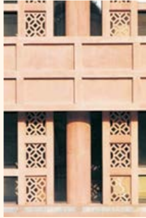
Jali panel by Raj Rewal's the Parliament Library at New Delhi, 2003 Source: http://ebuild.in/gallery/parliament-library
