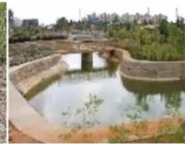
Rainwater Harvesting Ponds
