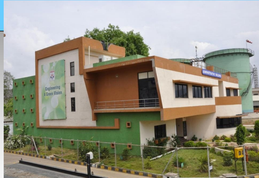
HPCL-Admin Building, Vizag
