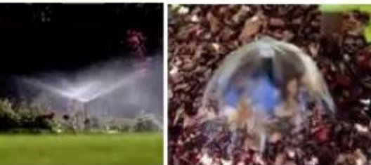
Efficient Irrigation System
