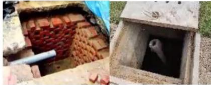
Rainwater Harvesting Pits
