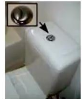
Dual Flush system with Low Flush rates
