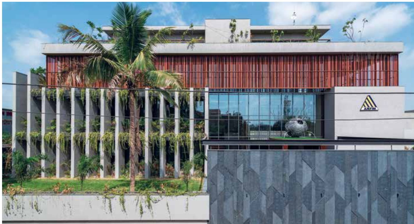
Figure 1: Street view of the building
