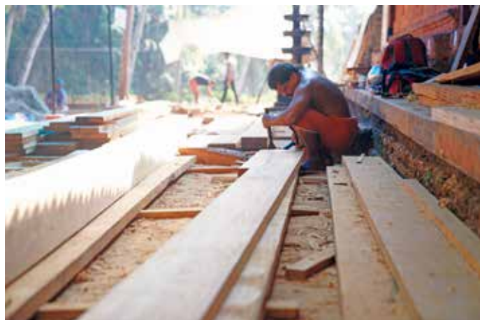
Figure 10: View of carpenter at work using Traditional Knowledge Systems
