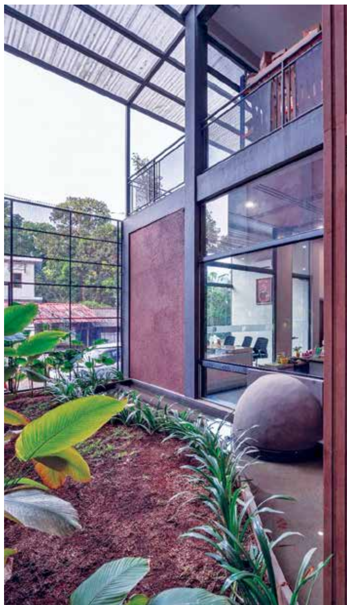
Fig 1: Courtyard with water body. Cooled air enters the office area through an underwater pipe.
