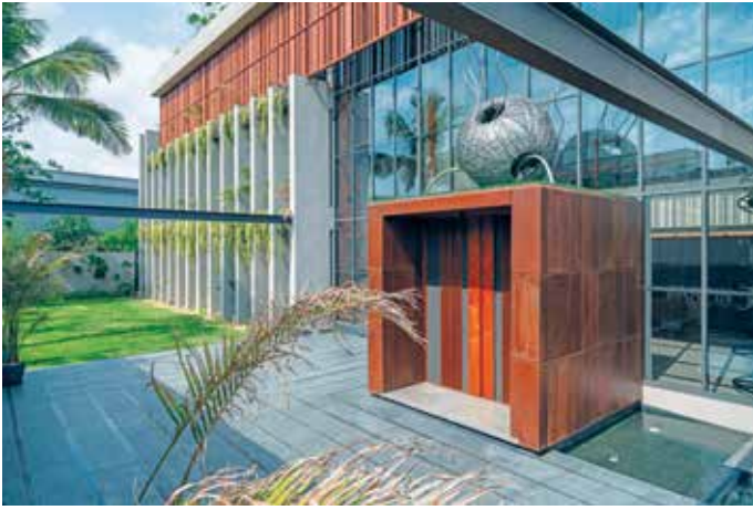
Figure 2: Entrance view of the building
