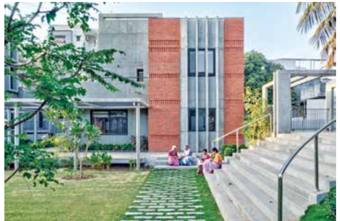
Fig 1: View From the Central Courtyard
