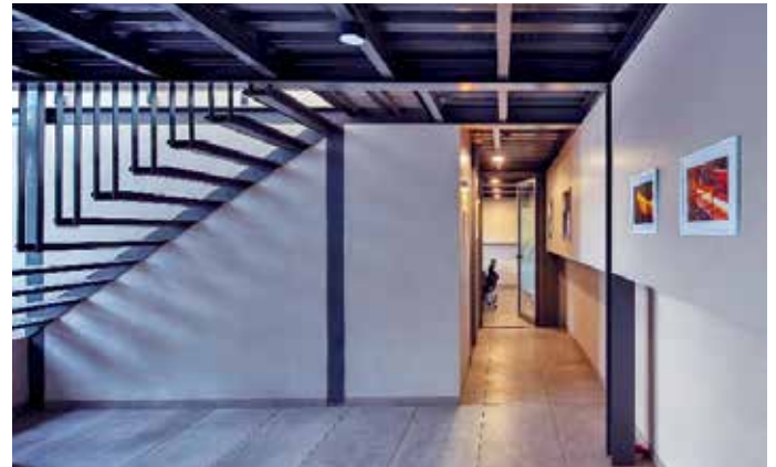
Figure 6: Intricate Details of the staircase and deck sheet slab, against the backdrop of simple interiors. Showcasing the ability and versatility of steel as a product. And its capacity to be solid yet flexible at the same time.
