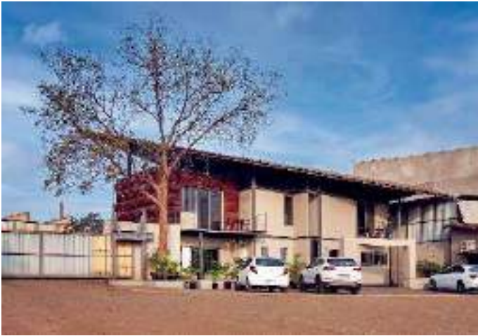
Figure 2: North east corner of the building with wall panels inserted into structural frames. The structural systems, as the aesthetics that showcase the clients products as well.
