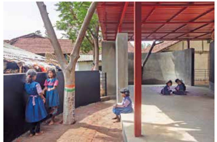
Fig. 6. The addition of semi-circular courtyards in the classroom was a response to enclose existing trees planted by students in the premises
