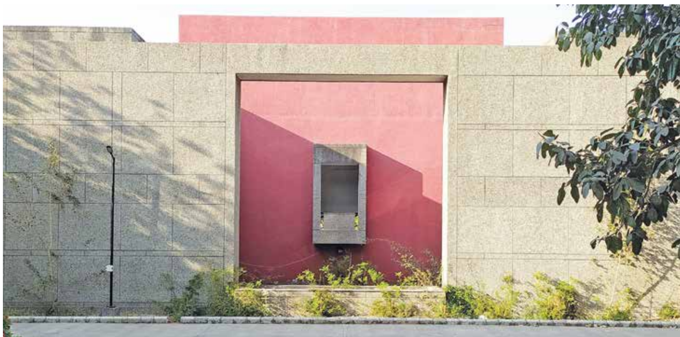
Figure 10: Southern and Western courts acting as light-wells
