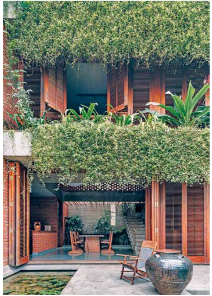
Figure 5: A series of louvred, sliding-folding windows which form a boundary between the enclosed and the al fresco, can control the connection in varying intensities.
