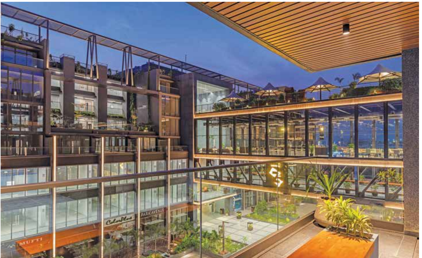
Figure 6: View of the connecting bridge from the viewing deck
