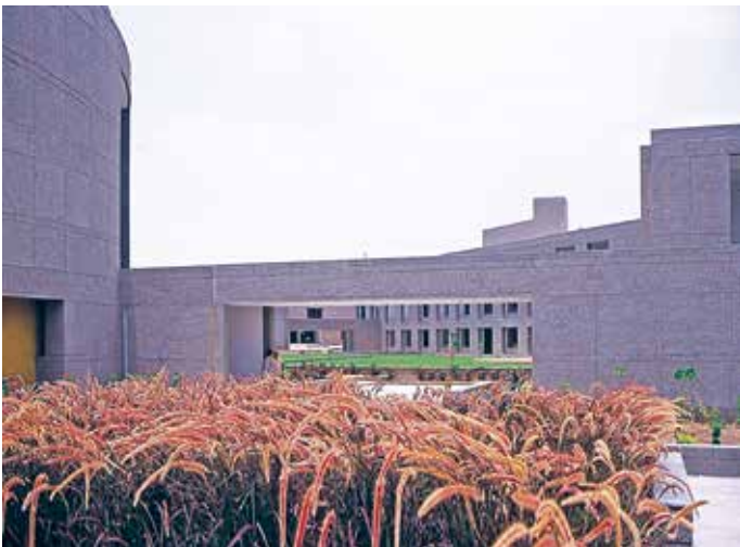
Figure 3: Entrance bridge as a Connector
