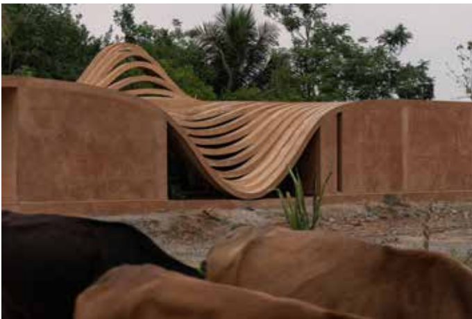
Figure 10: View from West Side
