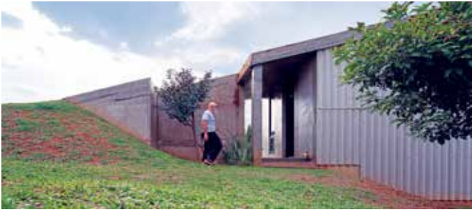
Fig 2 : Entry on East Side
