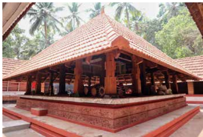
Figure 1: The restored Karnikara Mandapam at Kozhikode
