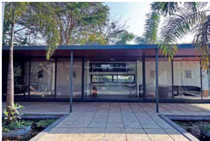
Fig 3: Sleek structural members supporting large overhang
