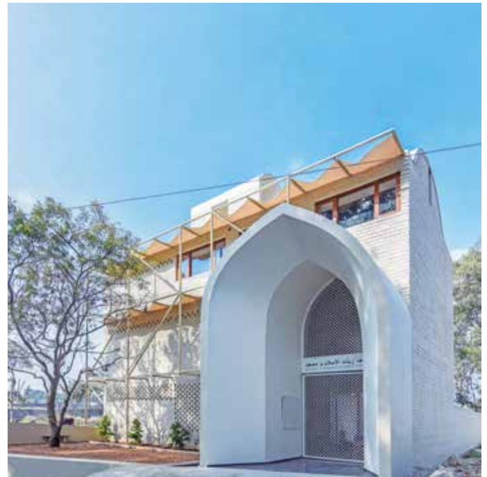
Figure 1: Main entrance (Frontage – Southern façade)
