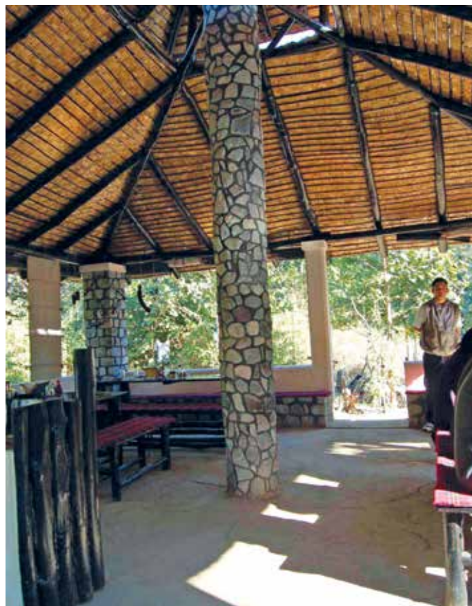
Figure 4: Truss System Made of Ballis (wooden poles) and Thatch
