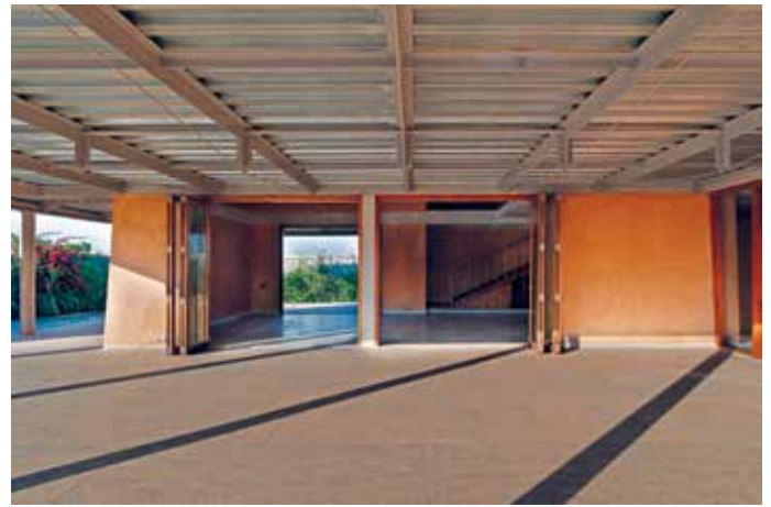
Figure 4: The Wrap around Verandah with a Light Weight Steel Roof
