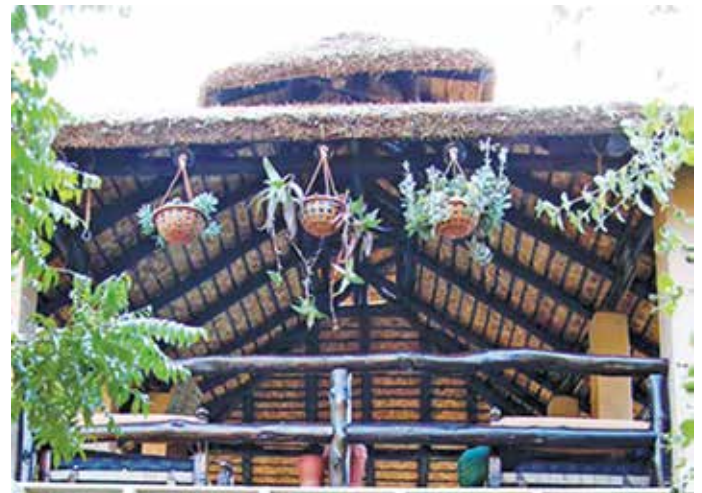
Figure 9: Upper Floor View of Machan
