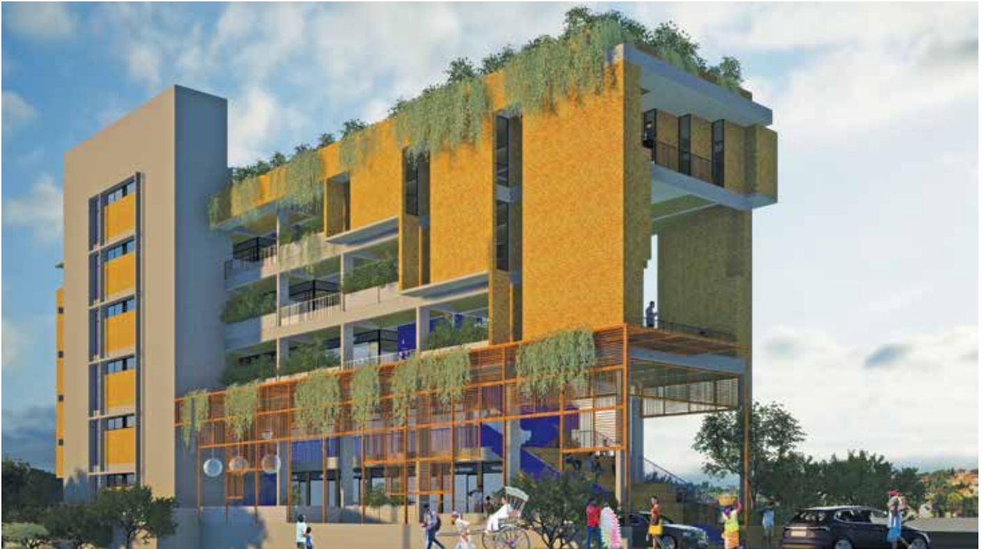
Fig. 9. West face with largely blank facades, recessed windows & bamboo screens with planting along with vertical circulation core.
