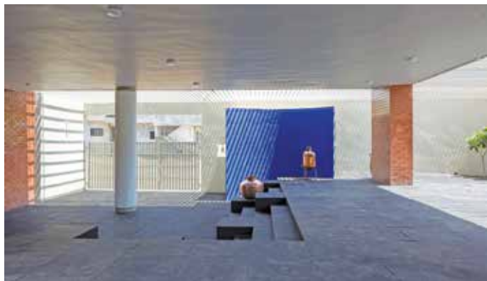
Figure 3: Entrance with security cabin
