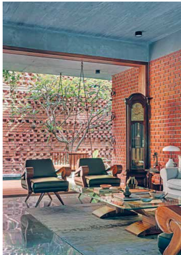
Figure 7: A long brick wall deployed parallel to the public zone behind a linear watercourt segregates the workspace from the home. Christened the 'dancing brick wall' by the architects, this load-bearing element features bricks laid in varying angles and different degrees of protrusion from the base plane, creating a perforated textural expanse whose three-dimensional beauty is further amplified by the sunlight that flows in from the skylight above. This was a strategic move, designed to facilitate ventilation between the work and home blocks without sacrificing privacy for the home. On its other side, lies a linear landscaped court brimming with greenery, another buffer zone to further separate the two areas.
