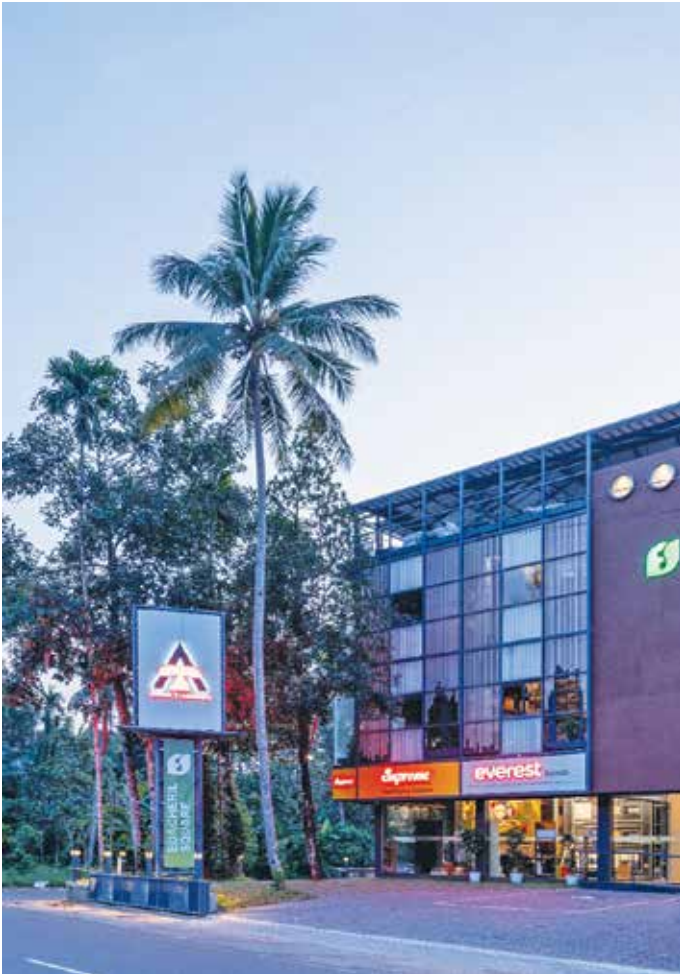
Fig 2: View from the street. Elevation with replaceable modular units made of materials being sold at the dealership and mud plaster over insulated ferrocement walls.
