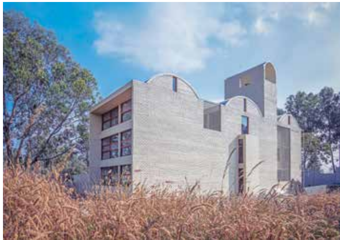
Figure 2: Rear (northern) façade
