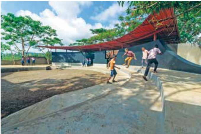
Fig. 4. The classrooms are covered with metal roof which goes along the curve of the wall, complimenting both the inside and outside spaces. The terracotta color of the roof merges with roof scape of the surrounding settlement
