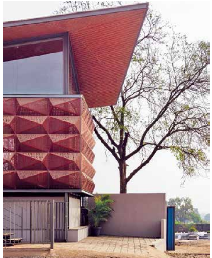
Figure 5: The scaling down of the mass by the vertical juxtaposition of the solid base at the bottom in bricks, translucent parametric metal screen & a completely transparent clerestory holding and lifting up the roof at the same time.
