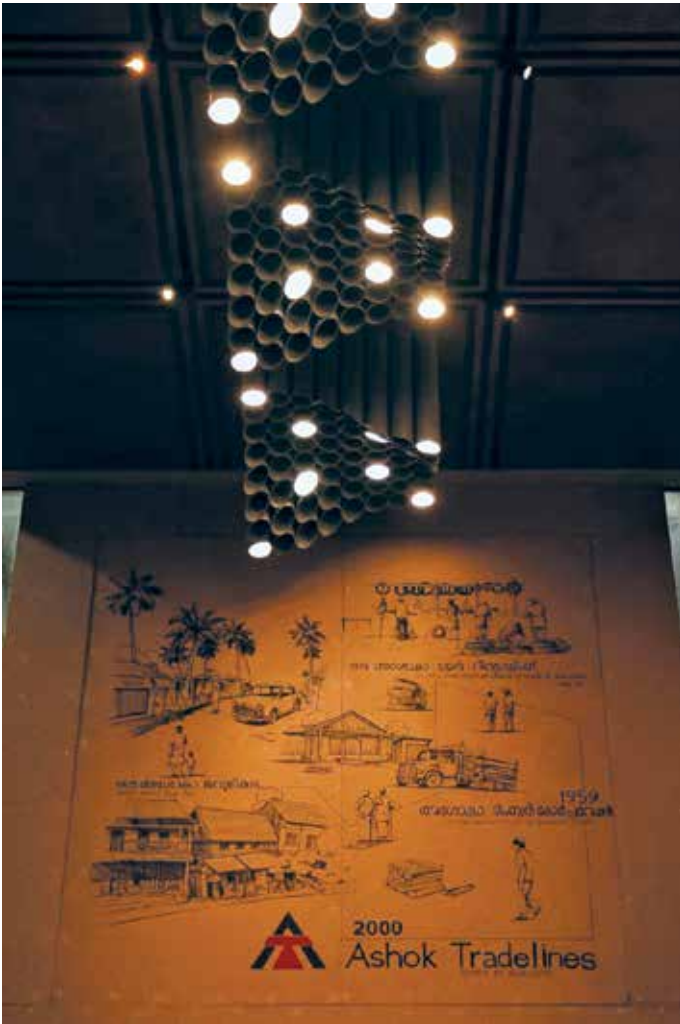
Fig 5: Custom-made ceiling light shades with waste PVC pipe cut pieces from dealership
