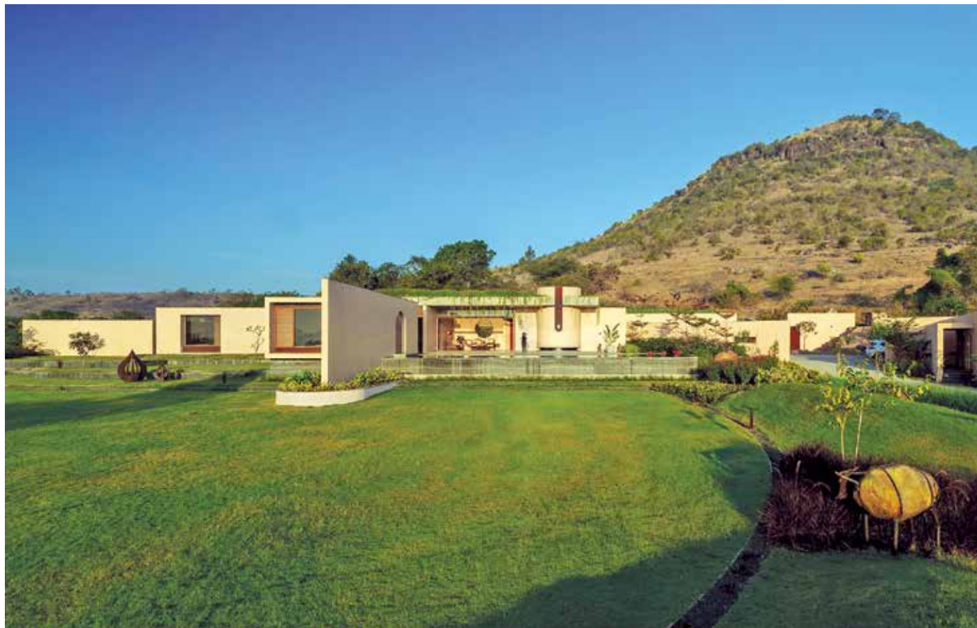
Figure 10: The gentle spacing of rooms breaks up the front elevation, creating a continuous interplay between public and private areas.
