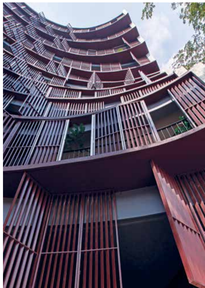
Figure 3: View showing curvilinear balconies opening into the tree courts
