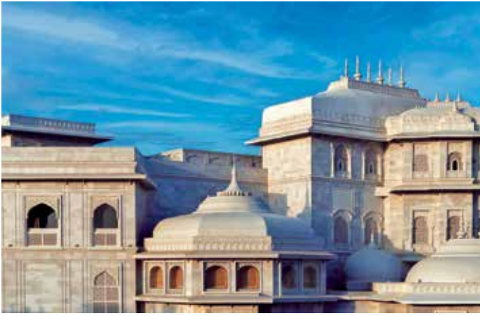
Figure 2: Rooted in heritage, the design captures the spirit of royal Rajasthan with domical roofs, layered façades and a hierarchy of spatial volumes.
