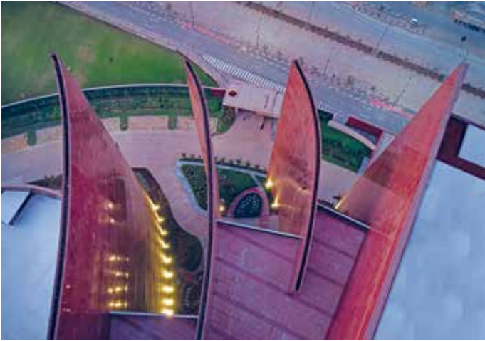
Fig. 7: High angle shot of the building's angular rooflines and red cladding.
