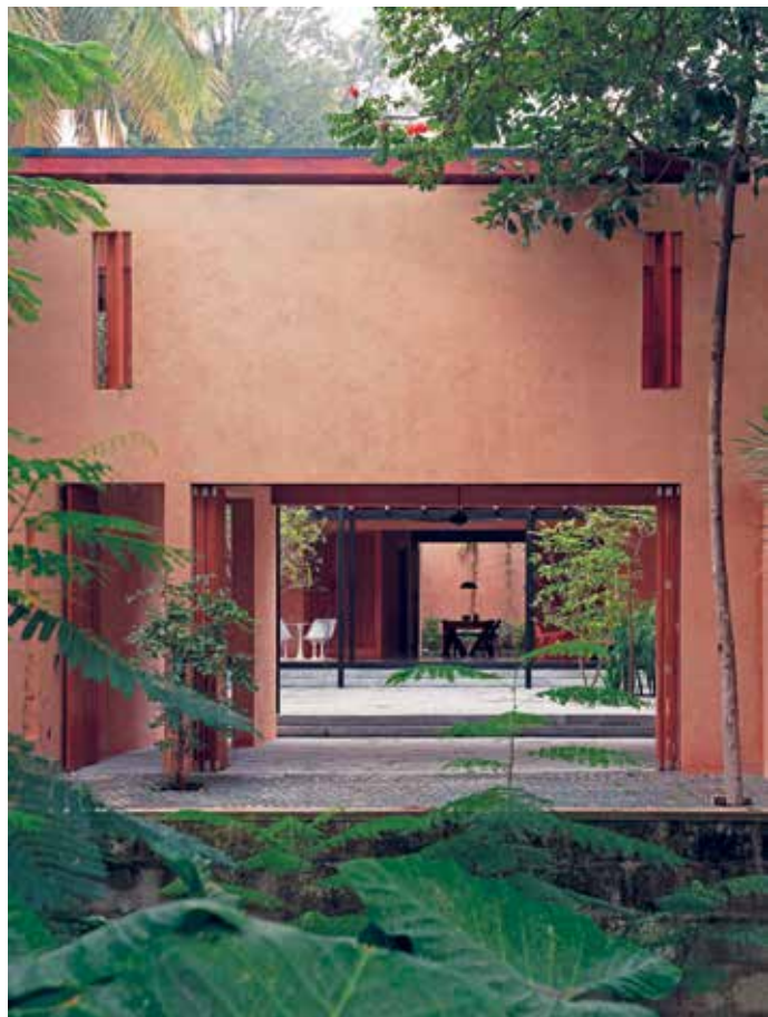
Fig. 1: View from the main entrance connecting a series of courtyards.
