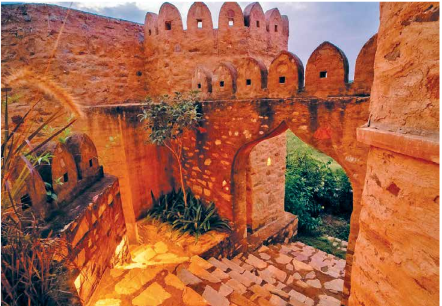
Figure 5: This image captures the enchanting entrance as dusk falls, the goal was to blend functionality with the rich narrative of historic architecture.
