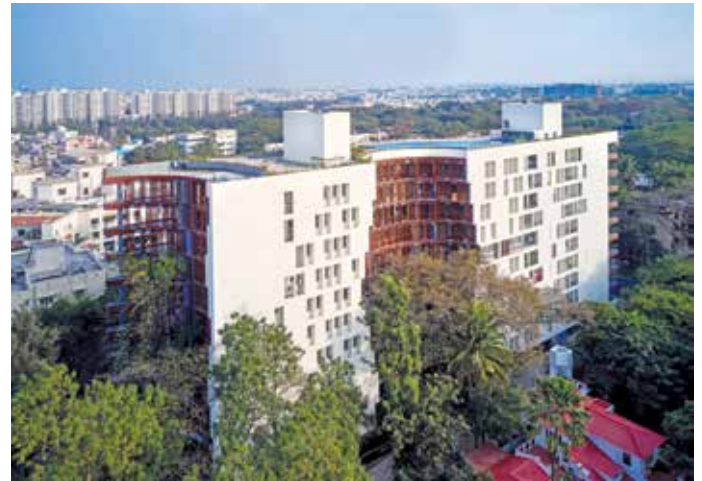
Figure 1: Aerial view showing how the building weaves around the trees
