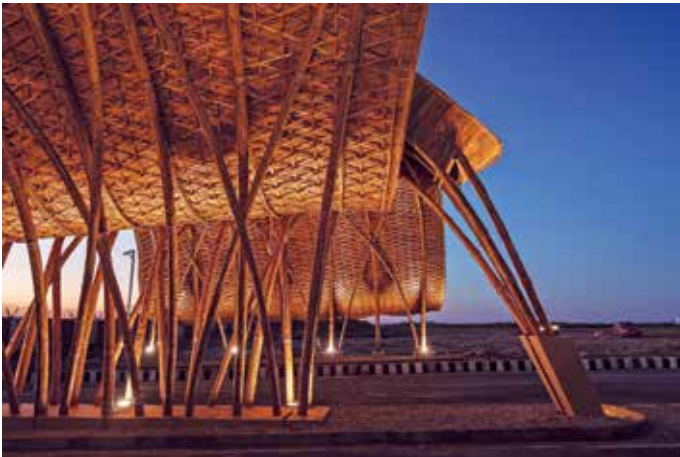
Figure 4: Some of the most striking characteristics of the Great Hornbill were incorporated into the design of the gate
