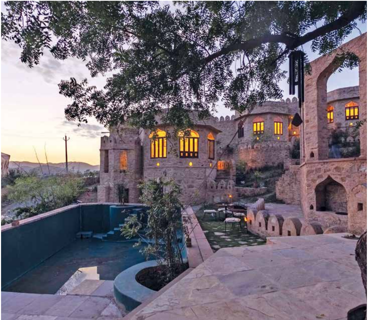
Figure 8: The pool, nestled within a carefully crafted catchment area, serves as a vital water body, collecting and managing all site runoff. This project not only enhances the aesthetic appeal but also promotes sustainable water management practices.
