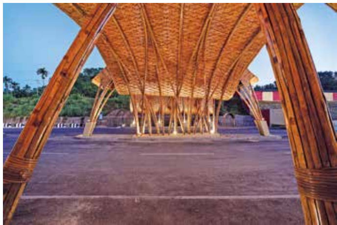
Figure 8: Covering an area of 2500 sq ft, the structure consists of 26 interlocking arches that form the wings of the majestic bird.
