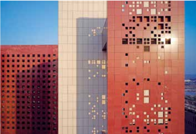
Fig. 8: Perforated sandstone and granite brise-soleil panels on the façade.
