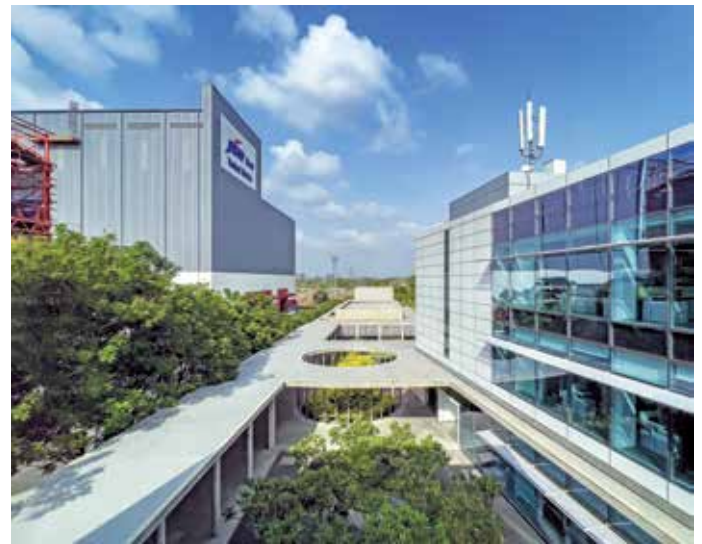
Figure 5: Courtyard seen from the connecting corridor at 1st floor. The office block resting over the unified base.
