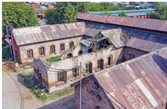
Figure 4: Drone image of Silk testing Building
