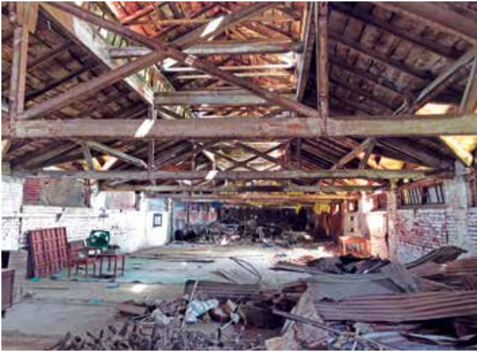
Figure 5: View of Filature building from inside
