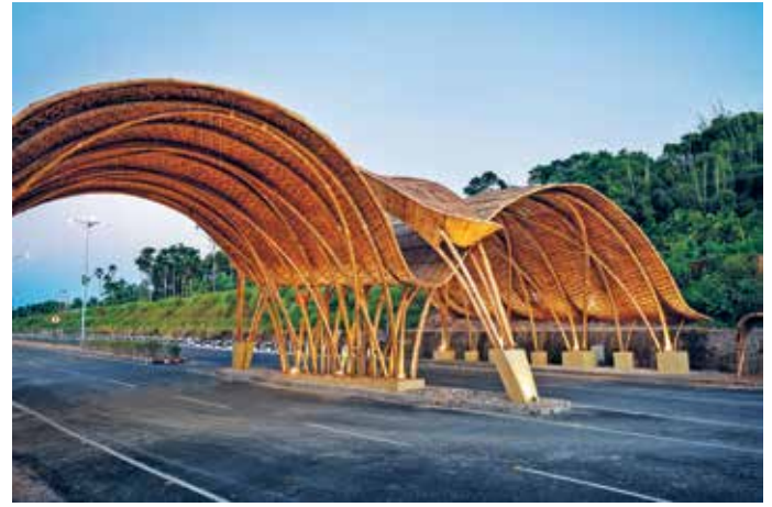
Figure 5: Redefining the utility of natural materials for traditional communities in the region, by building the structure entirely of bamboo and cane
