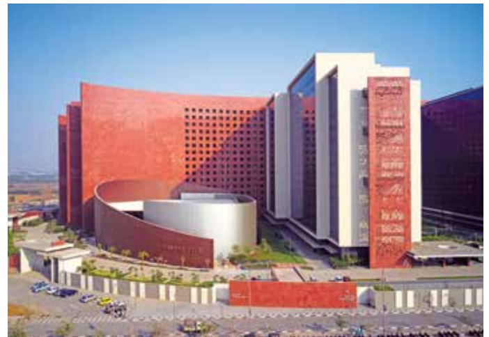
Fig. 5: Close-up of the façade materials: Lakha red granite and Gwalior white sandstone at the main entrance.
