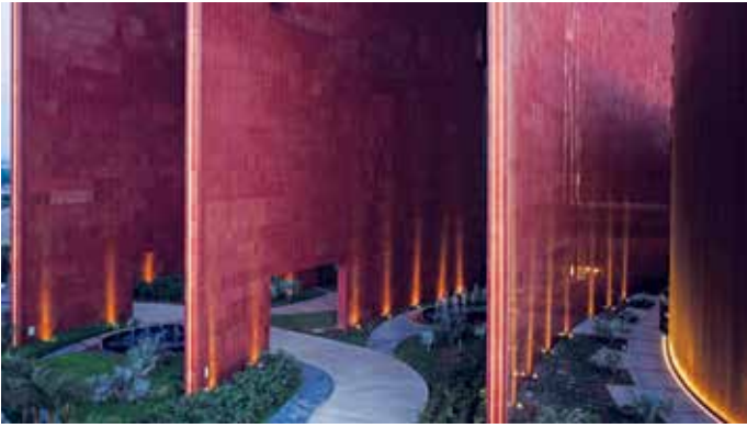
Fig. 6: Lakha red granite wall with adjacent shaded walkway and landscaping.
