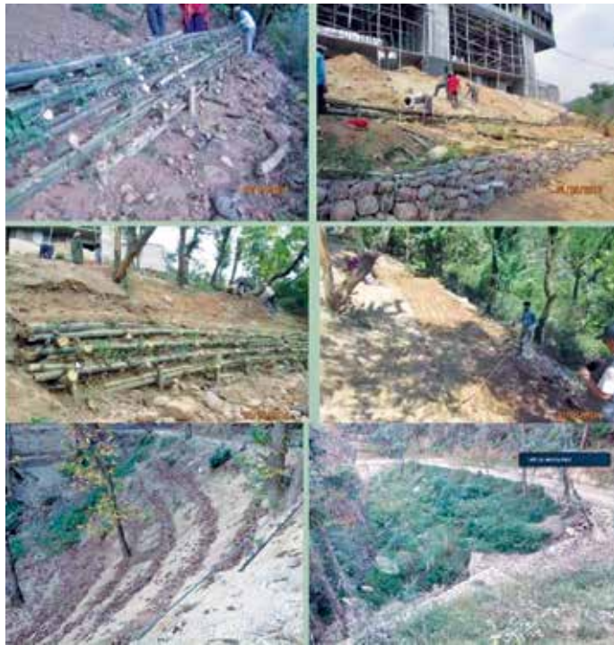
Figure 6: Bio Engineering techniques for soil stabilisation Source: Ar. Akshay Kaul workshop
