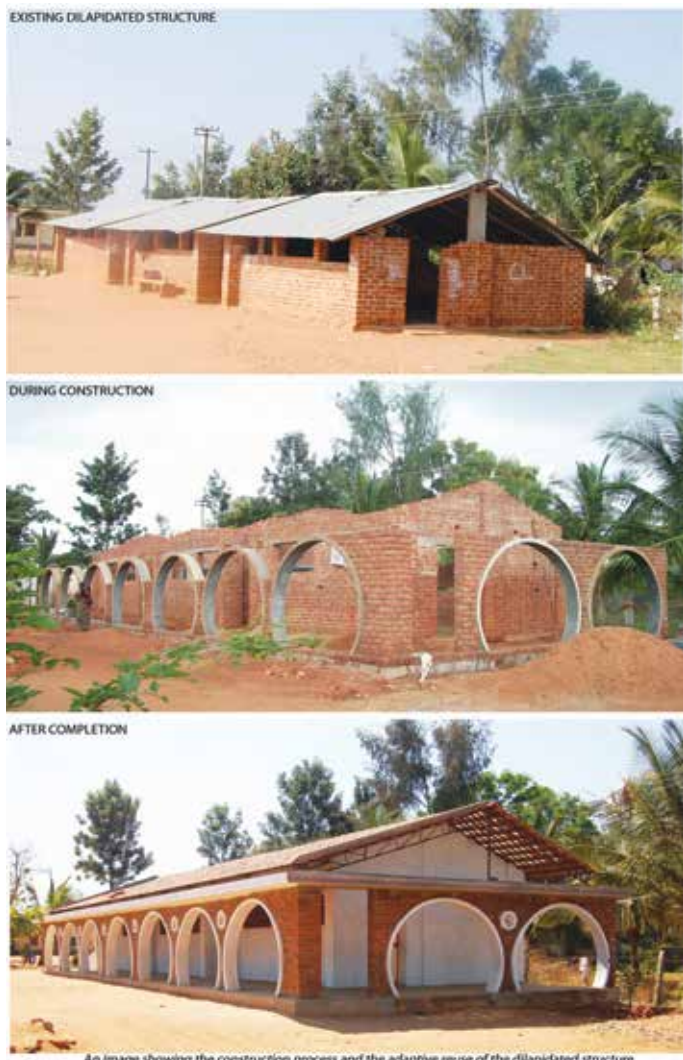
Figure 6: Adaptive reuse of dilapidated structure
