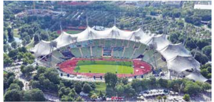
Figure 5: Olympia Stadium in Munich, Germany
