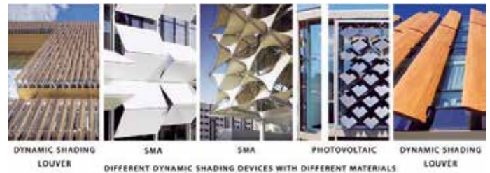
Figure 4: Different types of dynamic shading devices in different materials Source: Al-Yasiri & Szabó, 2021
