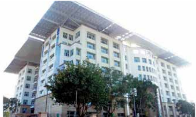
Figure 5: Building envelope of Indira Paryavaran Bhavan with 12m large overhang roof
