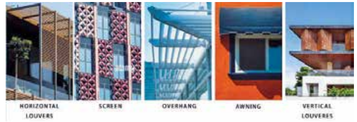
Figure 3: Different types of fixed shading devices in different materials Source: Kamal, 2010
