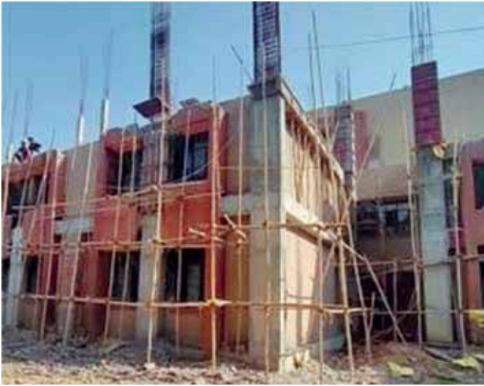
Fig. 4: Showing Exoskeletal structure growing around the existing building
