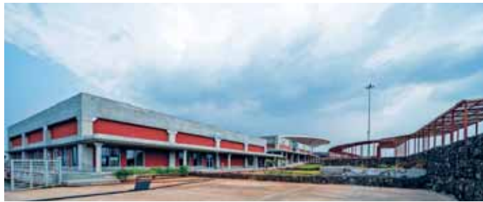
Figure 9: Usage of Murum in plinth
