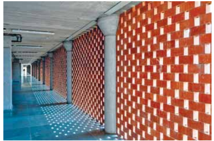
Figure 8: Brick jali for filtered sunlight
