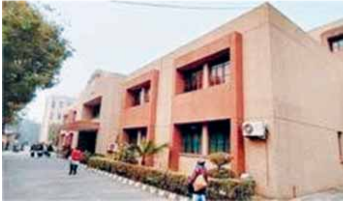
Fig. 1: Showing the existing Building of Fr. Agnel School, Greater Noida
