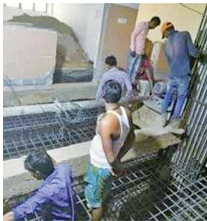
Fig. 3: Showing Retrofitting of foundation and re-strengthening of column
