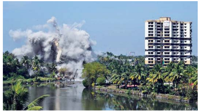
Figure 1: The Golden Kayarolam apartment at Maradu being demolished in January 2020 Source: The Hindu , September 26, 2021
