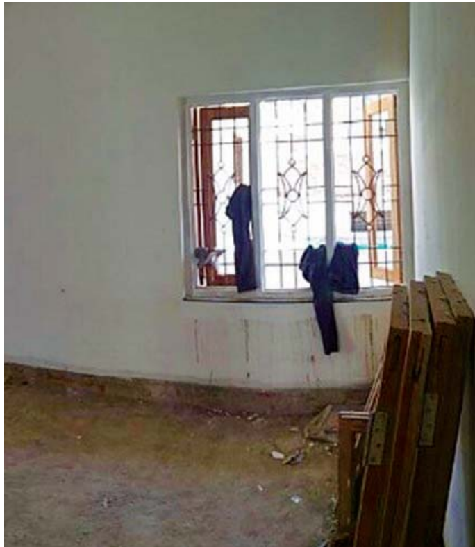
Figure 4: Interior View of Existing Room
