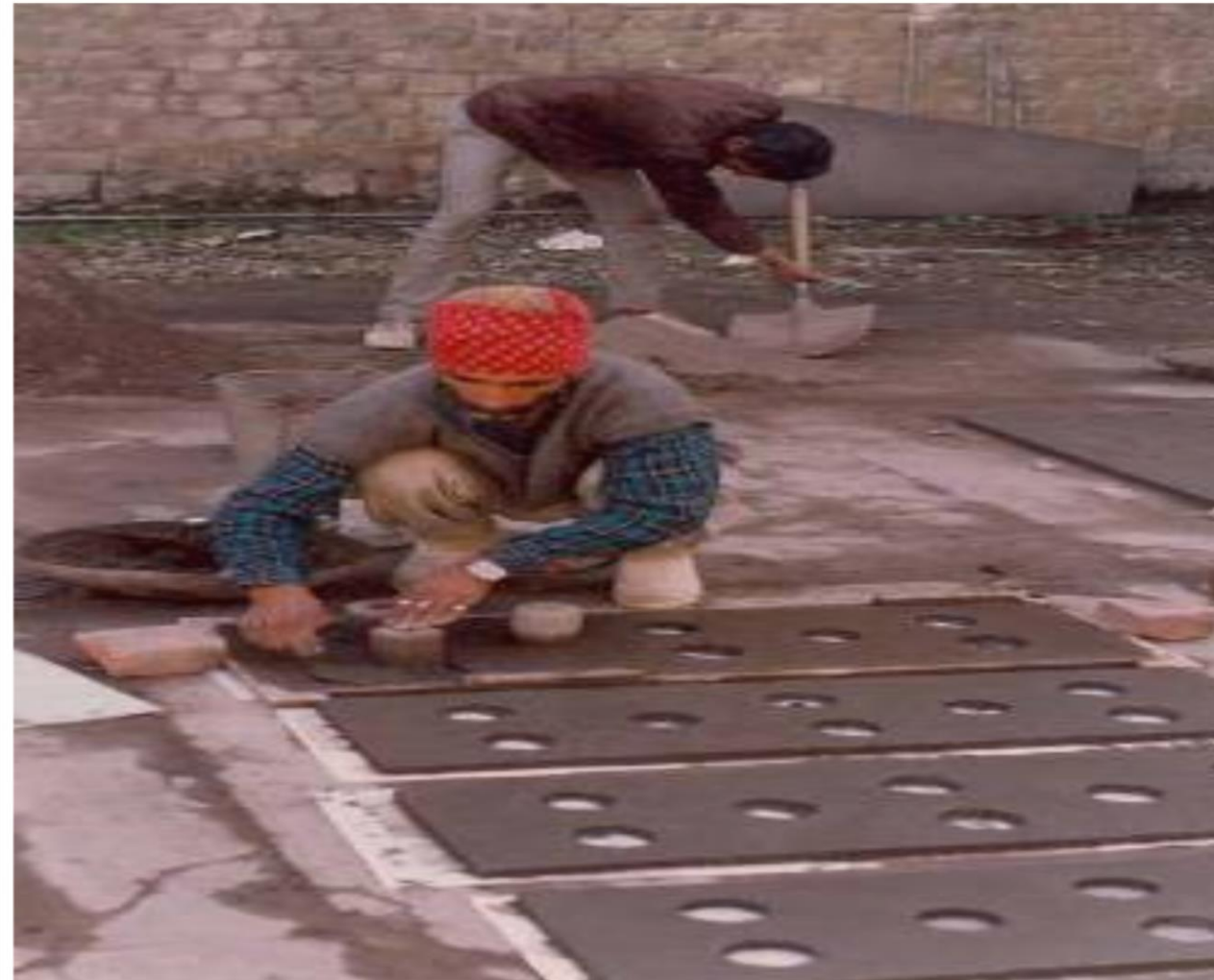
Construction of Ferro-cement Columns and Slabs
