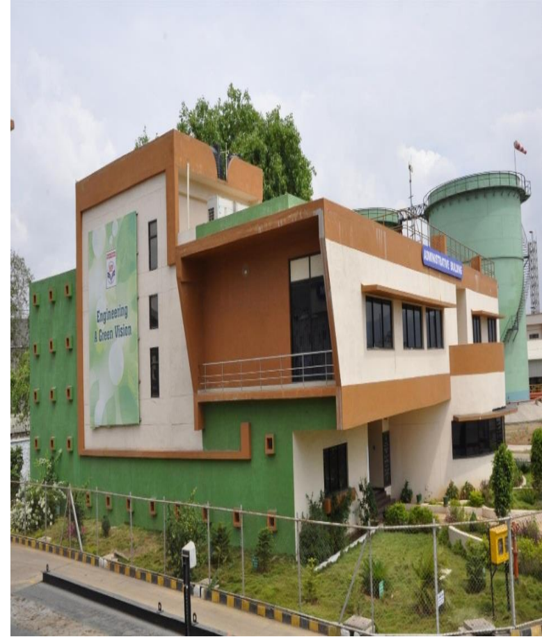
HPCL-Admin Building, Vizag
