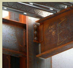
Double Angle Connection
