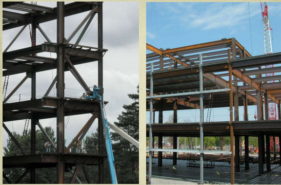
braced frames (left) and rigid frames (right)
