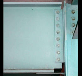
Partially-Restrained (PR) Connections
