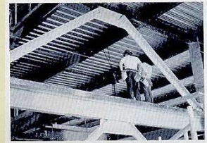
Figure 4.16 Inverted K bracing with double-angle connections.
