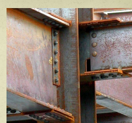
Bolted Flange Plate Connection
