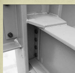
Welded Flange Plate Connection
