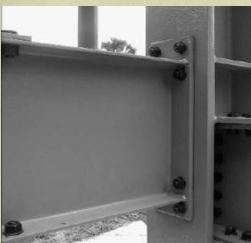
Bolted Extended End-Plate Connection
