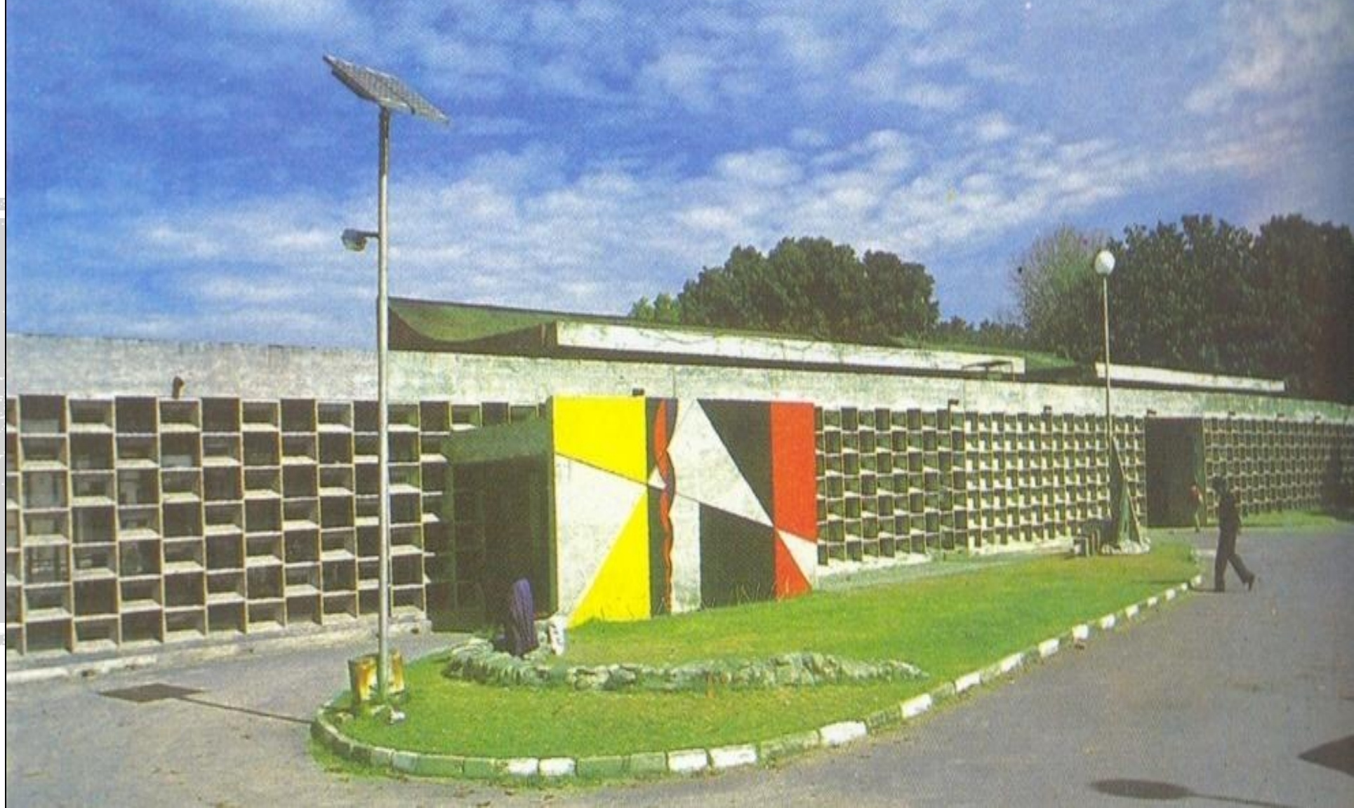
COLLEGE OF ARCHITECTURE FRONT FAÇADE ADORNED WITH DEEP SCREEN OF PRE-CAST CONCRETE, A SORT OF MINIATURE brise-soleil
