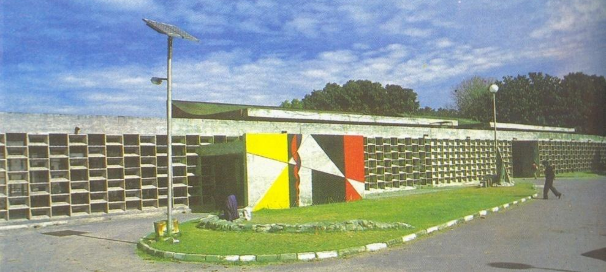
COLLEGE OF ARCHITECTURE FRONT FAÇADE ADORNED WITH DEEP SCREEN OF PRE-CAST CONCRETE, A SORT OF MINIATURE brise-soleil
