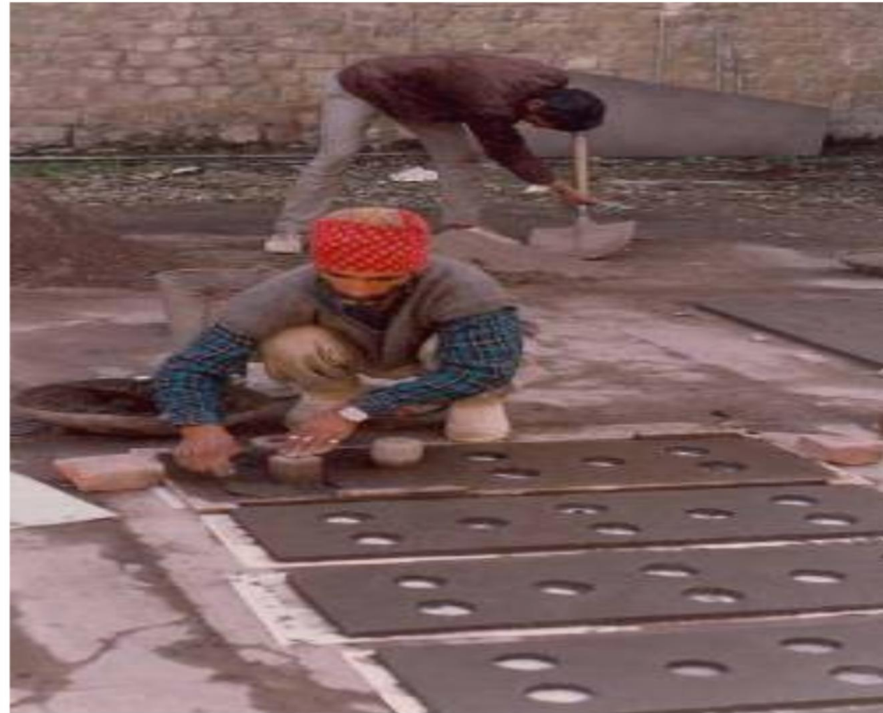
Construction of Ferro-cement Columns and Slabs
