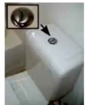
Dual Flush system with Low Flush rates
