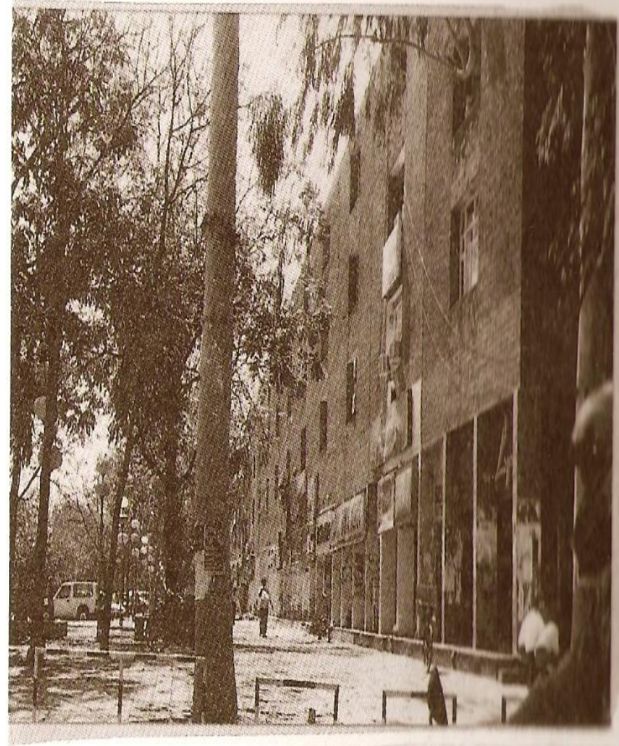
Straight and uniform brick block with rectangular concrete column recessed balconies on upper floors.
