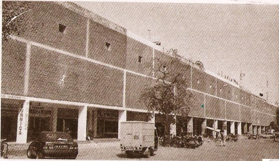
Blank façade in exposed brick work without any decorations. Only concrete bands have been provided to break the monotony.
