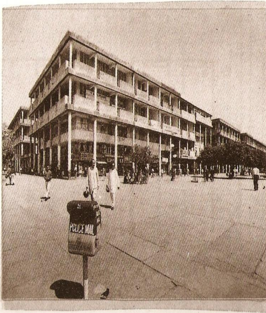
An unending view of RCC structures with uniform skyline in the city-centre.
