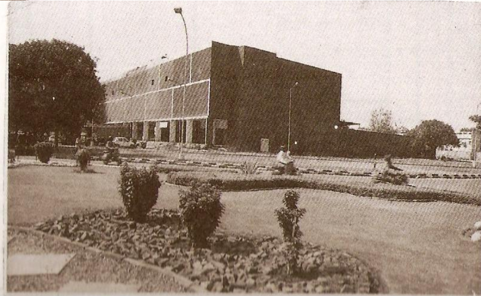
Side elevation of a showroom with courtyard boundary wall at the back
