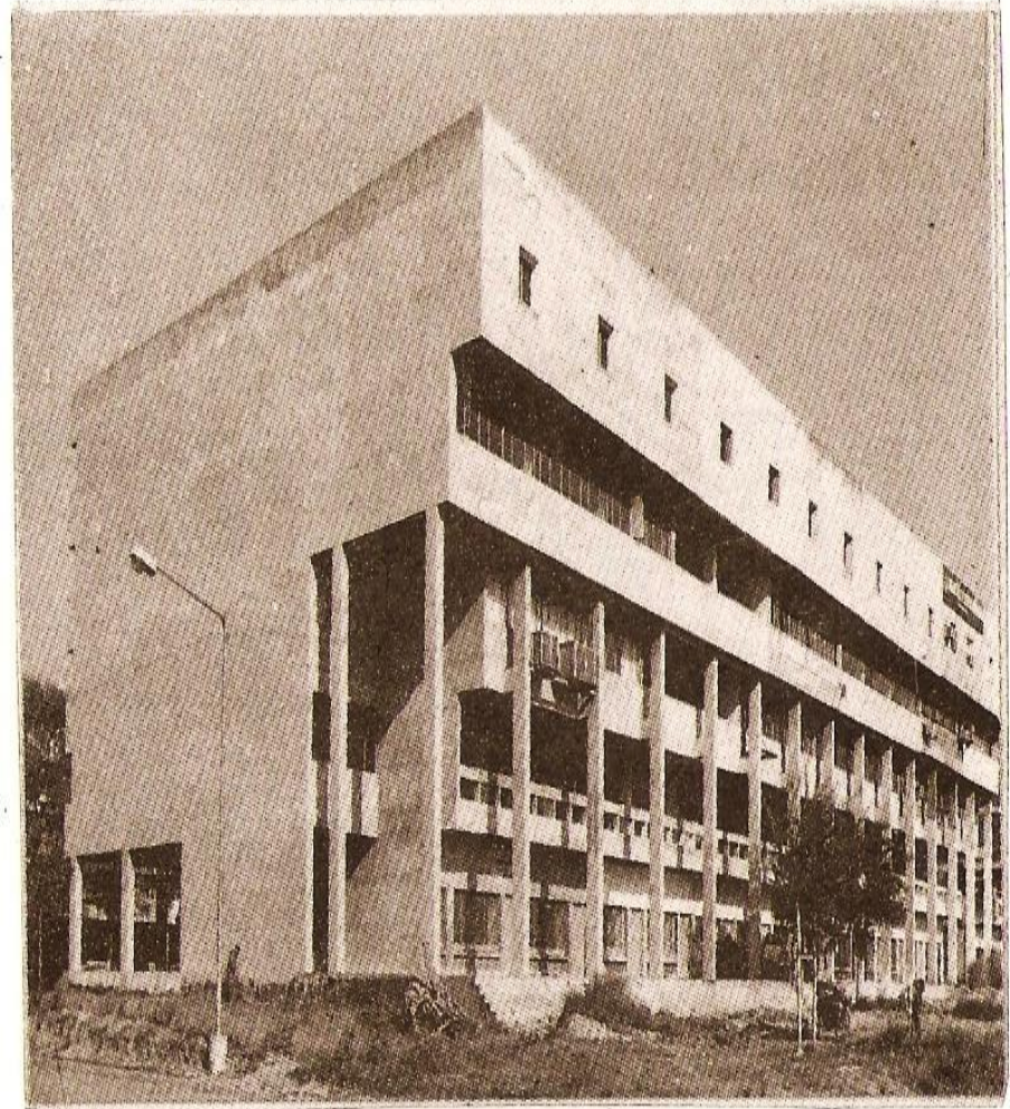
Shop-cum-offices in the sub-city centre built in exposed RCC work without plastering or colour wash.
