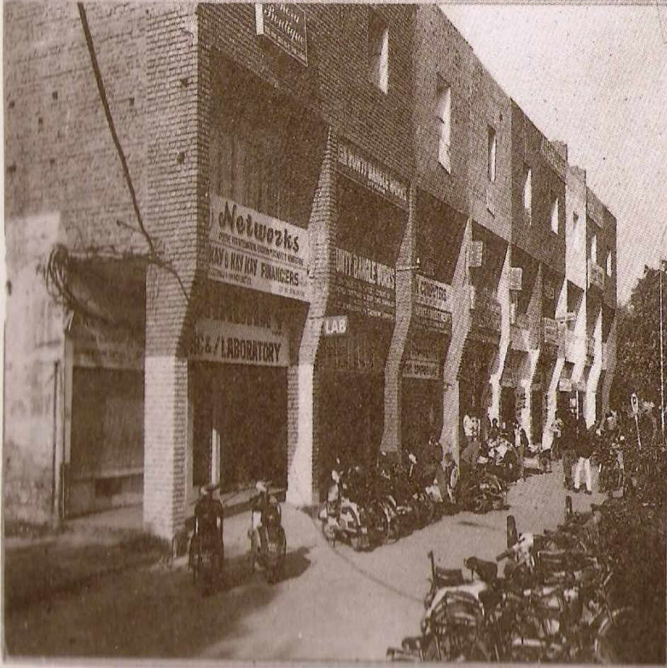
Front view of shop-cum-offices in exposed brick work and corbelling in the pillars.
