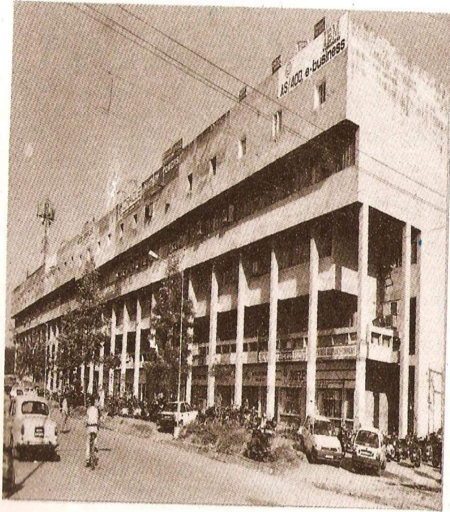
Upper floors are projecting over previous floors, increasing the depth of floor space.
