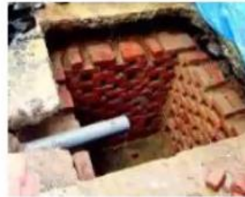
Rainwater Harvesting Pits
