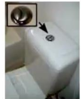
Dual Flush system with Low Flush rates
