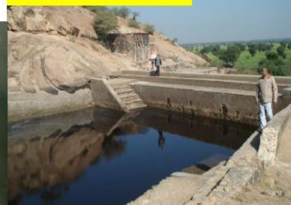
Rain Water Harvesting
