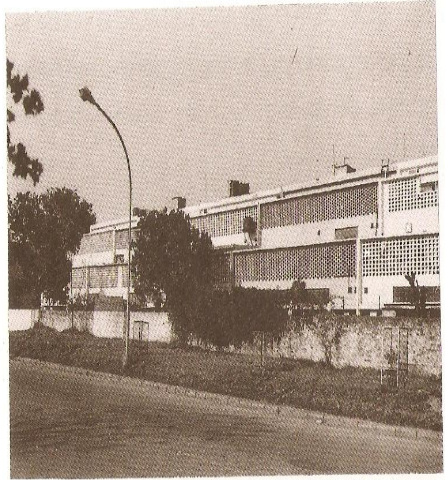
Rear view of 10-marla houses with standard design of brick jallis (New control has relaxed this control)
