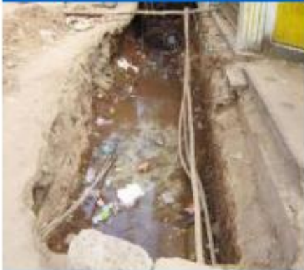
Storm water drains
