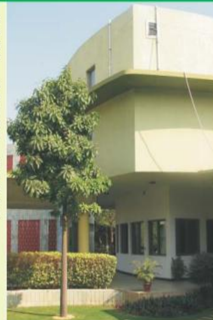
The inner courtyard of the building
