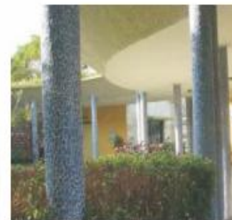
Salvaged tiles for pillar cladding
