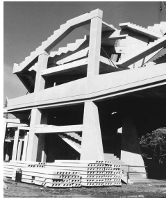
Uniquely shaped structural elements for a sports stadium
