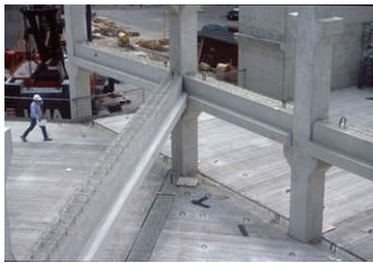
Inverted Tee beams supported Precast columns on precast columns
