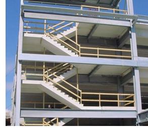
Precast concrete Stairs
