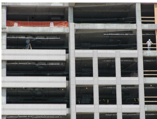
Precast Concrete Cladding
