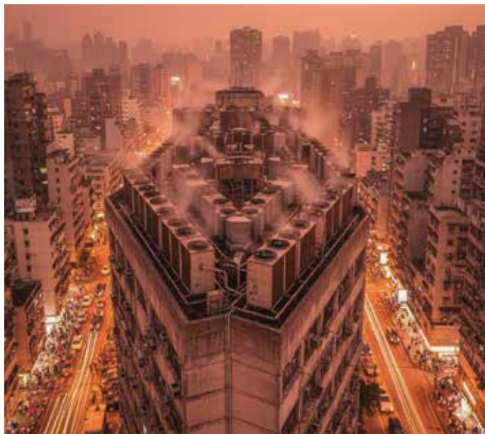
Figure 2: Visualisation of outdoor AC condenser units in a dense urban setting
