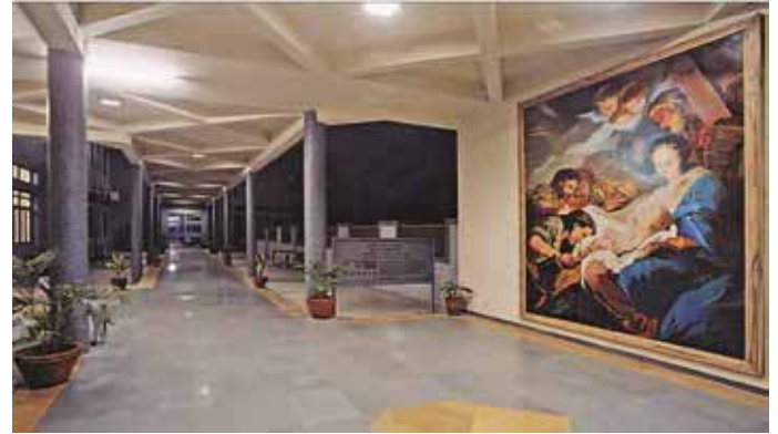
Fig 5: Mother and Child Centre, Miraj – Diagonal beams
