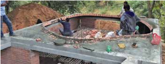
Fig 6: All 4 corners meeting to form a complete course, dome taking a fish-eye form Source: Kakani Associates
