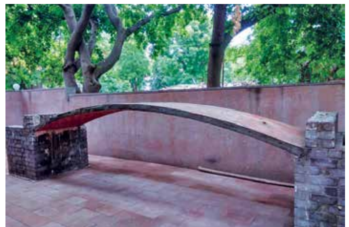
Fig 10: Layer 4 to complete the vault of 80mm thickness Source: Kakani Associates
