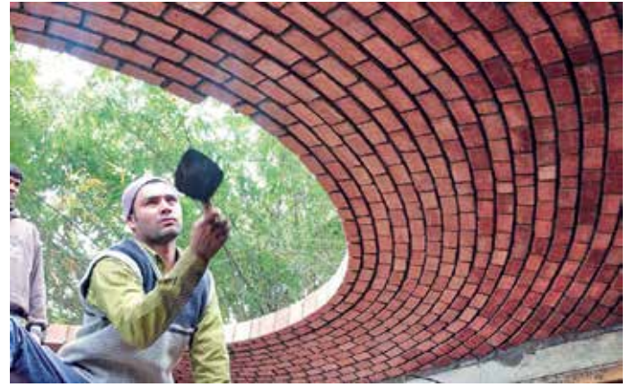
Fig 2: Master craftsman Azad Singh constructing the shallow dome in Alluva, Gandhinagar
