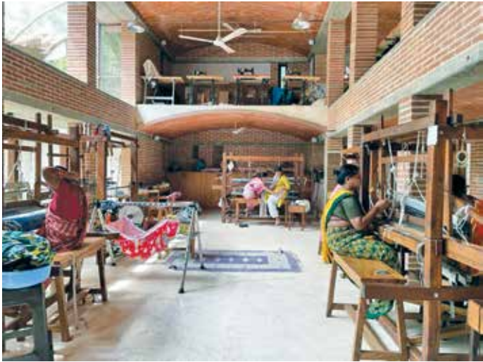
Fig 12: The completed 4.75m span vault at SOACH NGO Source: Kakani Associates
