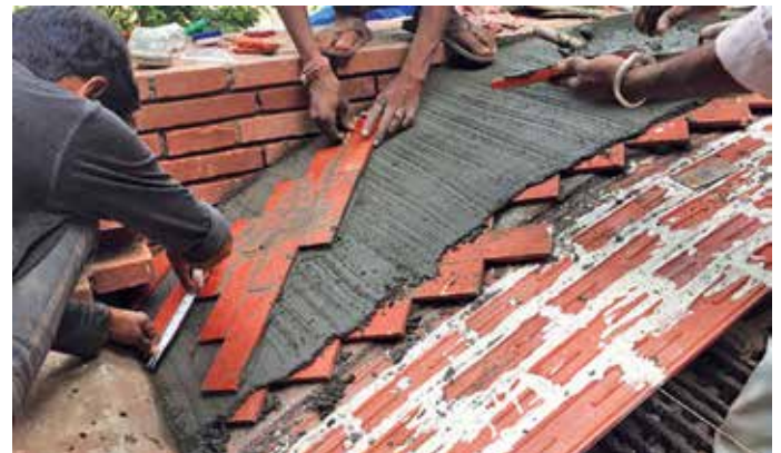
Fig 9: Construction of the 3m span vaults at SOACH NGO Source: Kakani Associates
