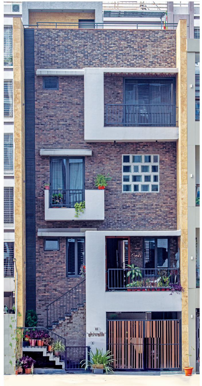
Figure 1: Front Facade facing east direction
