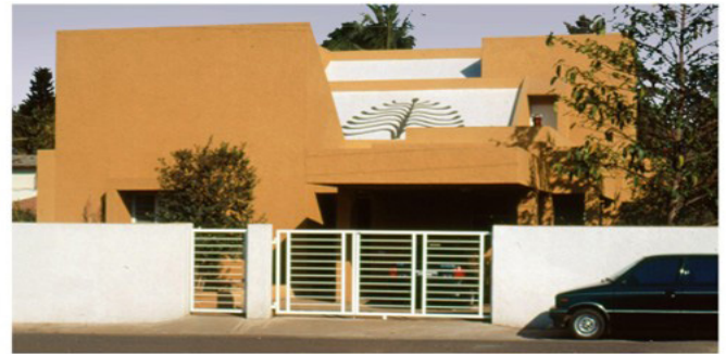
Image 9: Brock House- External view
