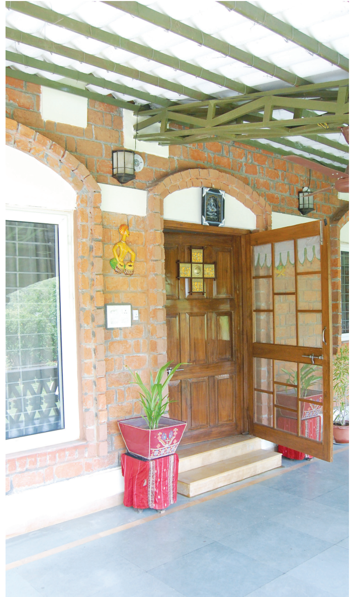
Figure 12: Entry door with steel frame
