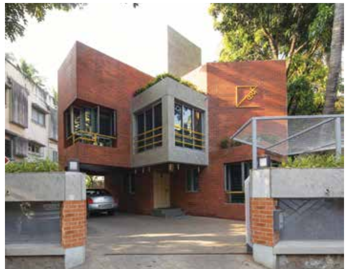
Image 9: View from the street after renovation
