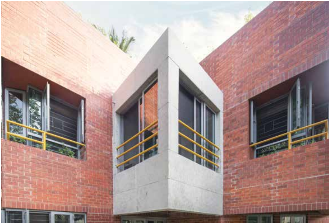
Image 1: A view of the renovated Karna Bungalow, with its protruding blocks and unconventional angles.
