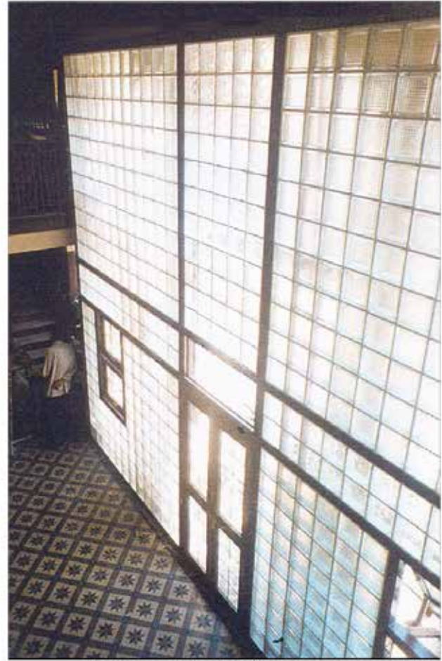
Roadfront verandah enclosed for protection from noise & dust Added in 1999 - Architect Harshad Bhatia
