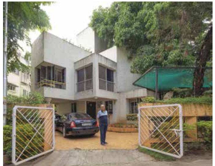
Image 8: View from the street before renovation
