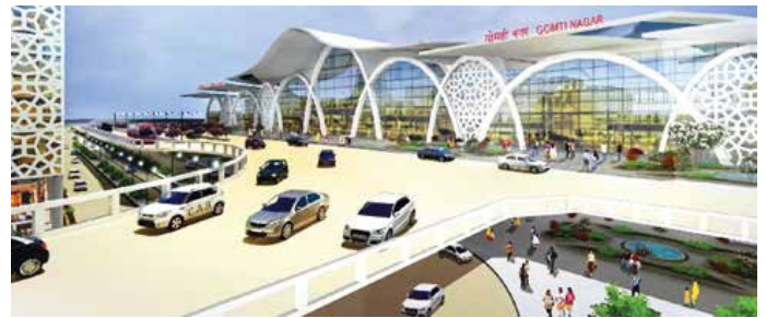
Figure 7: Gomti Nagar Railway Station in Lucknow
