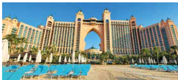
Figure 1: The imposing structure
