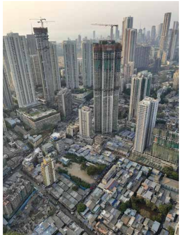
Figure1: Aerial view of Mumbai high rises under construction. Source: Shutterstock
