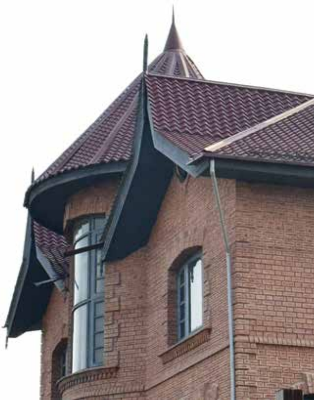
Figure 4: Exterior view showing the conical roof
