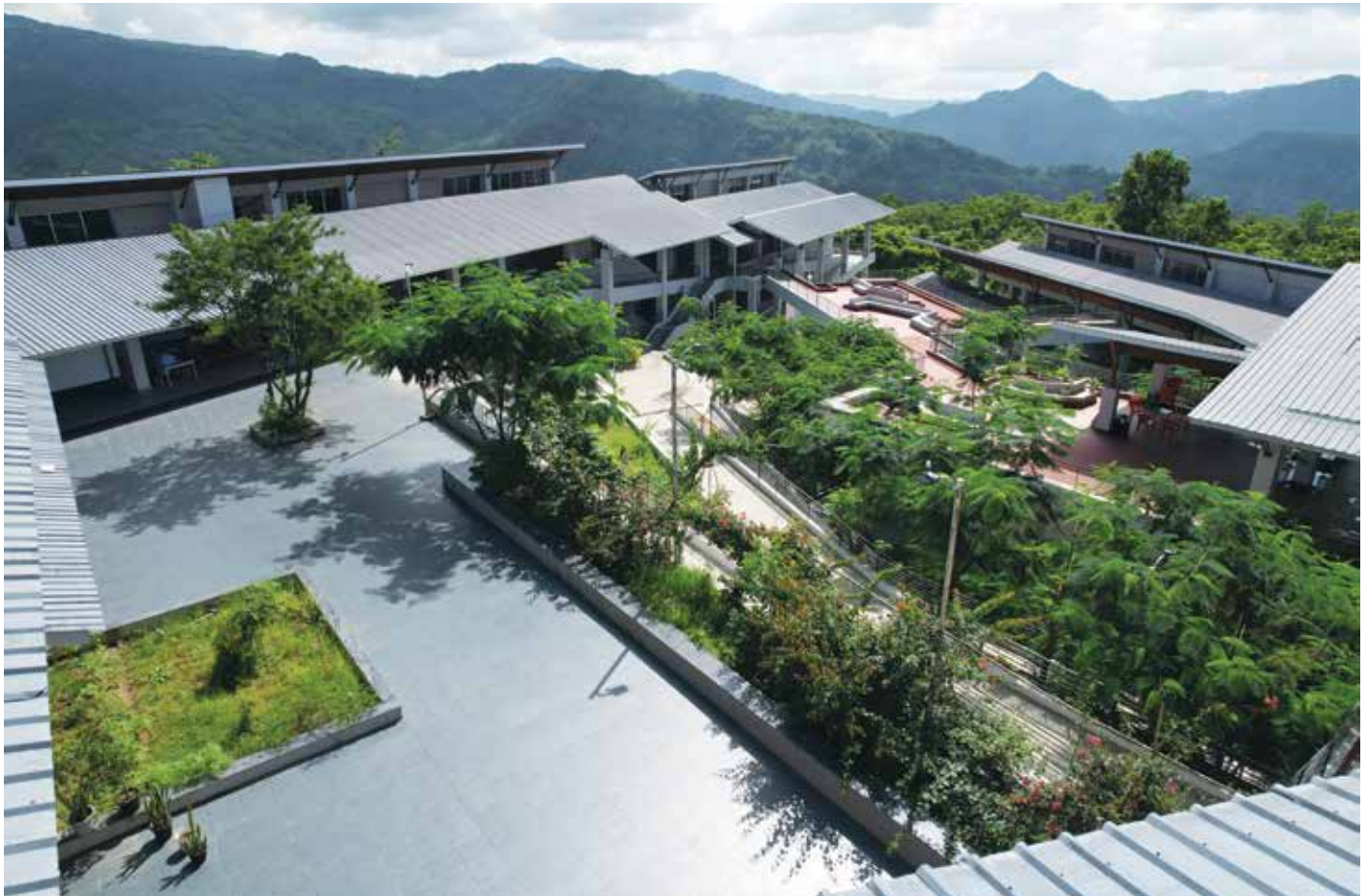
Figure 1: View from faculty block. Stepped courts unify the blocks and blocks are kept low to allow views of the distant mountains.
