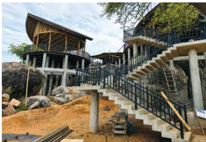
Figure 4: Elevated Walkways and Pavilion Structures The Visitor Information Centre under construction, with elevated stairways, timber pavilions and concrete supports carefully positioned around the existing rock formations, demonstrating how the design adapts to the natural terrain while maintaining a strong architectural character.
