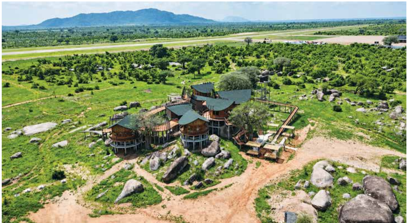
Figure 1: Aerial View of the Visitor Information Centre
