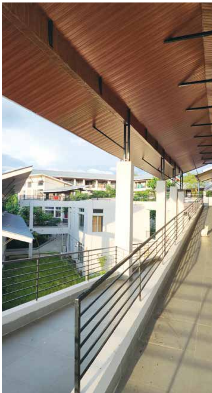
Figure 5: Ramps run along the verandah and connect the blocks and courtyards
