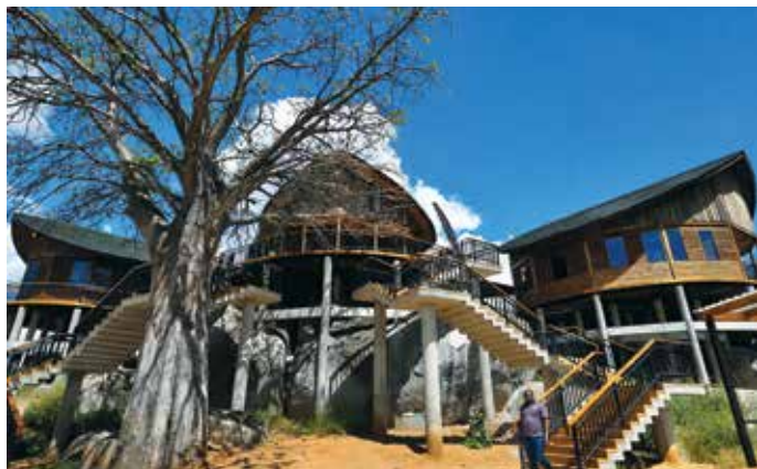
Figure 5: Main Front view and Elevated Structures The Visitor Information Centre rises above natural boulders, using timber, concrete columns and raised walkways to respond respectfully to the existing terrain.
