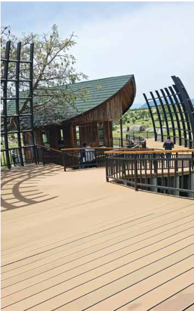
Figure 10: Timber Deck and Viewing Platform
