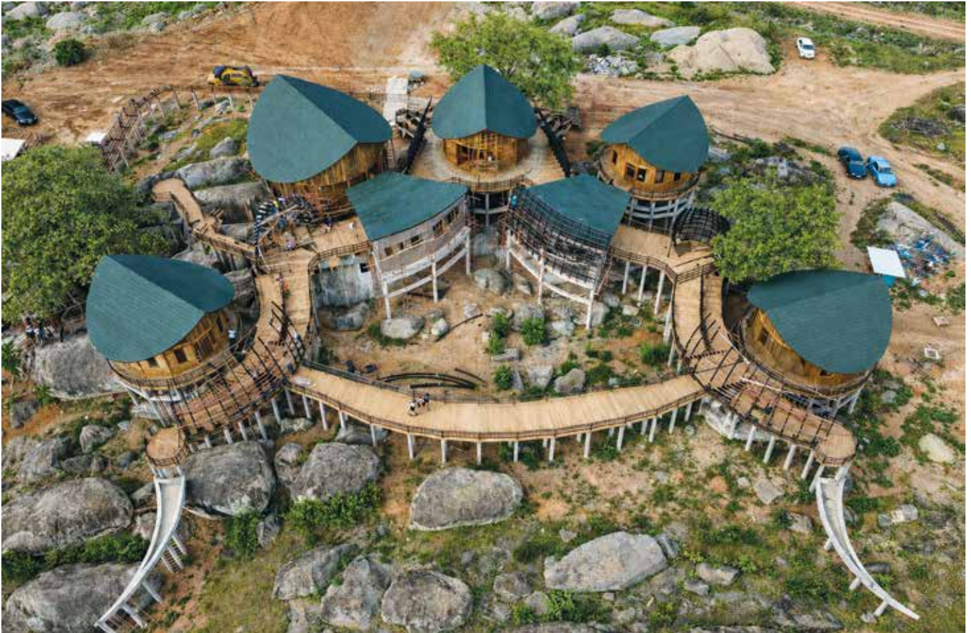
Figure 2: Aerial View of the Visitor Information Centre
