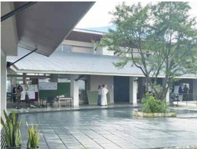
Figure 7: Deep verandahs and overhangs offer outdoor jury spaces even in the monsoon rains (Block A).
