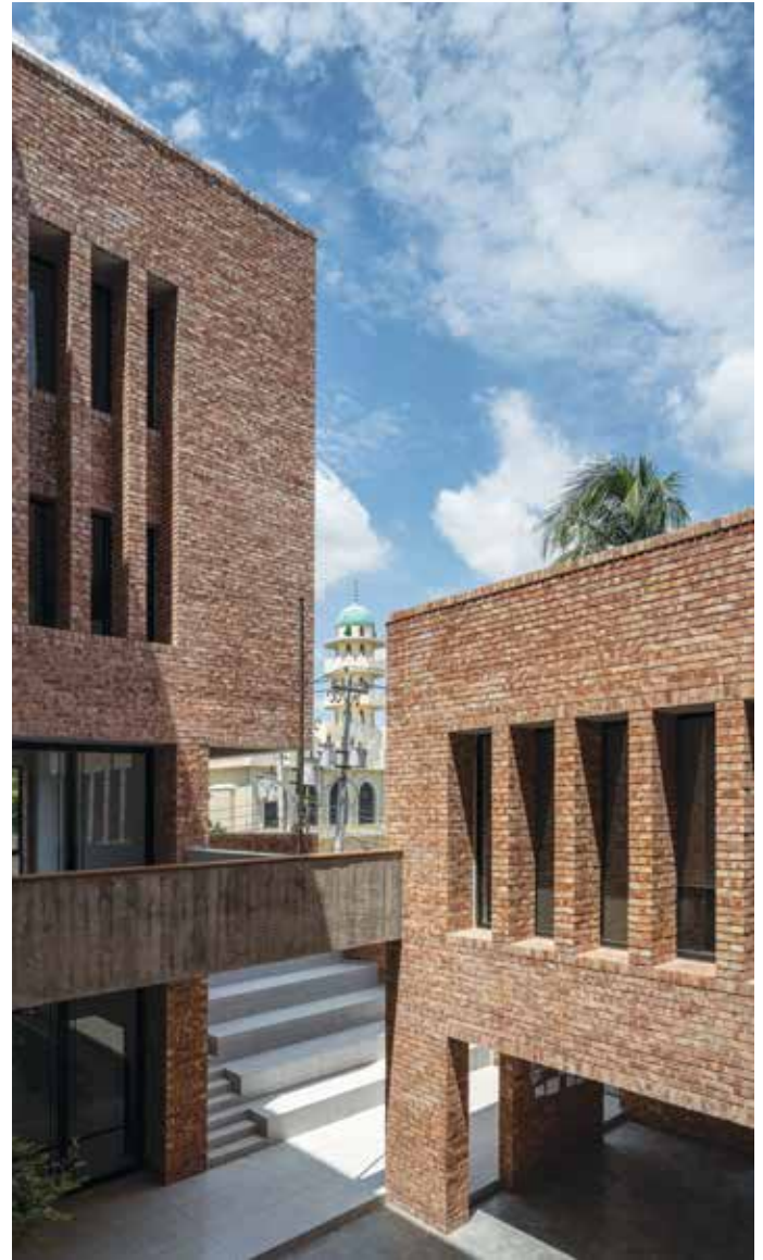
Figure 6: View from Internal Courtyard towards Social Stair
