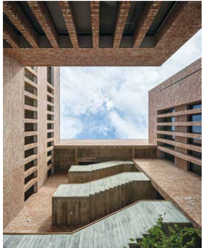
Figure 3: Open to Sky Central Courtyard
