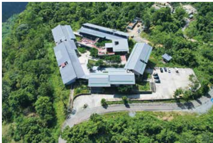
Figure 2: Aerial view from SE showing the wooded surroundings. Main approach from the university hub is from the south.
