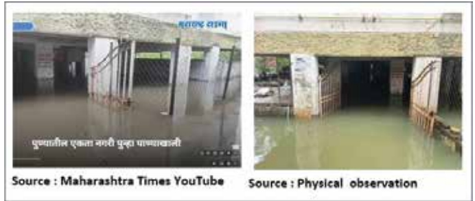
Fig. 8: Flooded Parking Source: As mentioned
