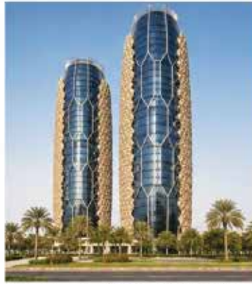
The twin towers with a dynamic facade inspired by traditional mashrabiya.
