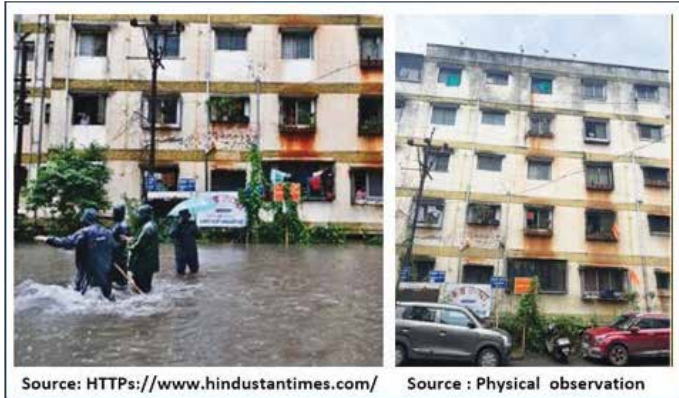
Fig. 7: Flood affected upper floors Source: As mentioned
