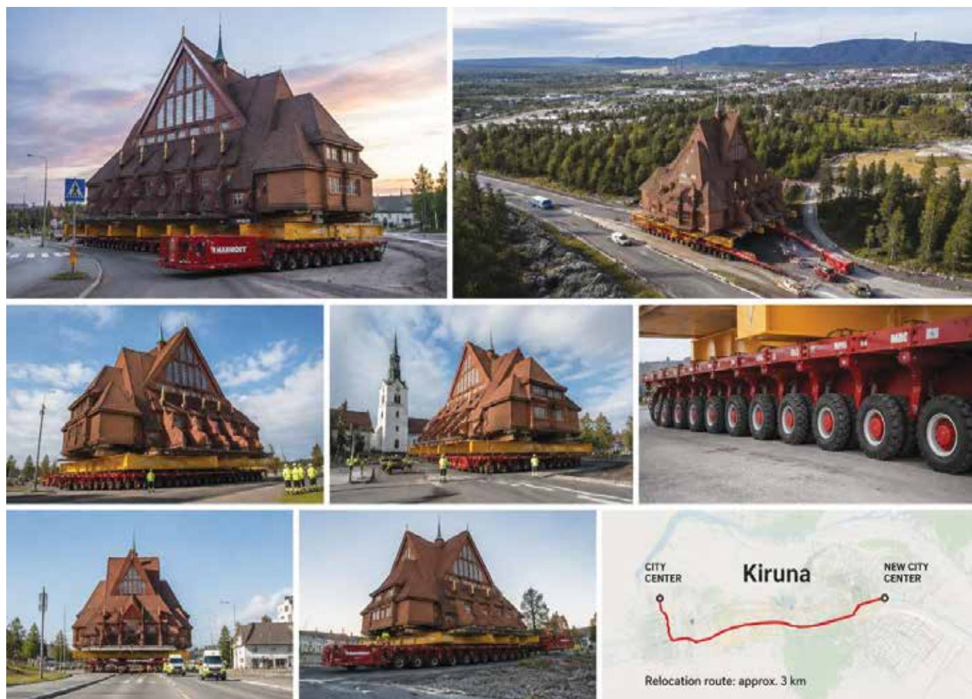
Figure 10. Relocation of Kiruna Church, Kiruna, Sweden
